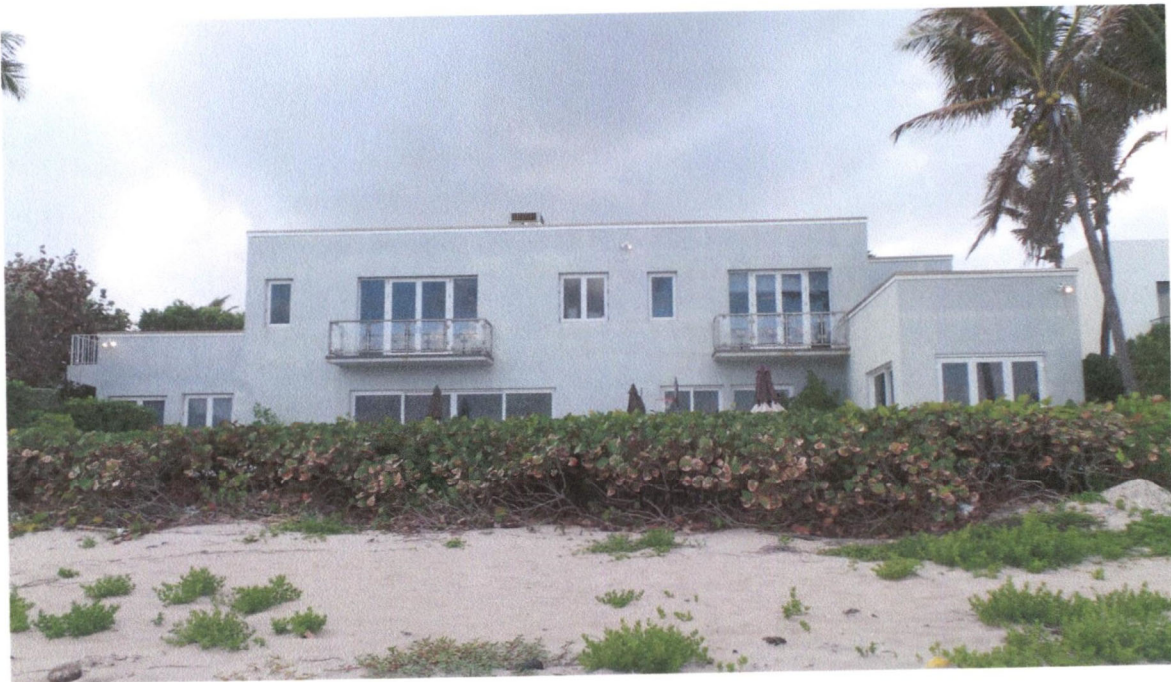
Rear (East) Facade
