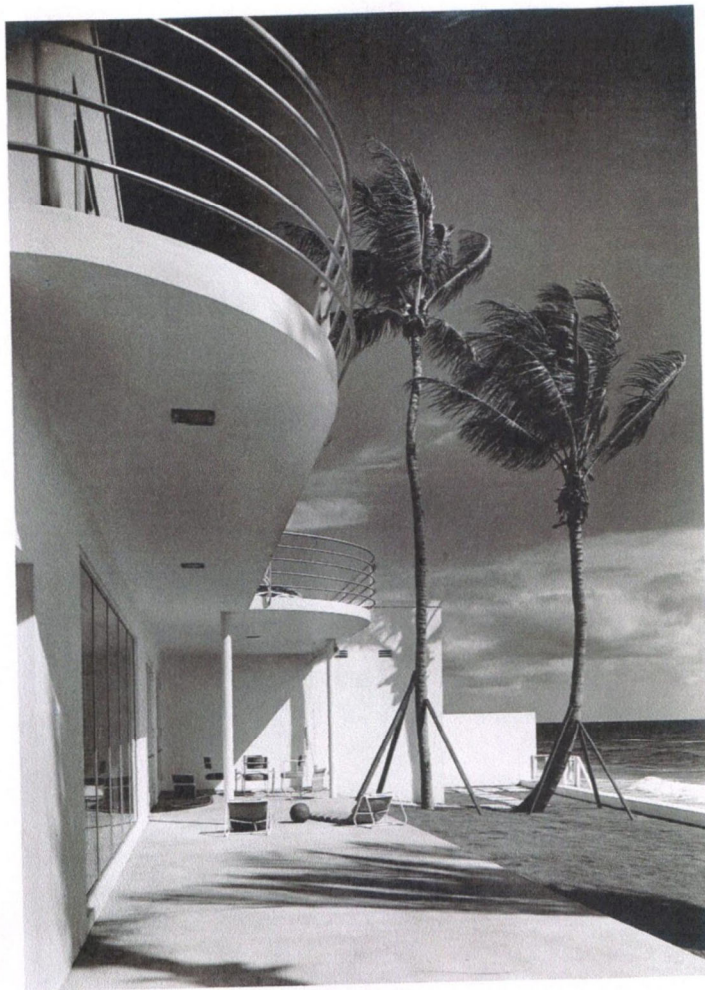
Rear (East) Façade with Curvilinear Balcony Courtesy of the John L. Volk Foundation
