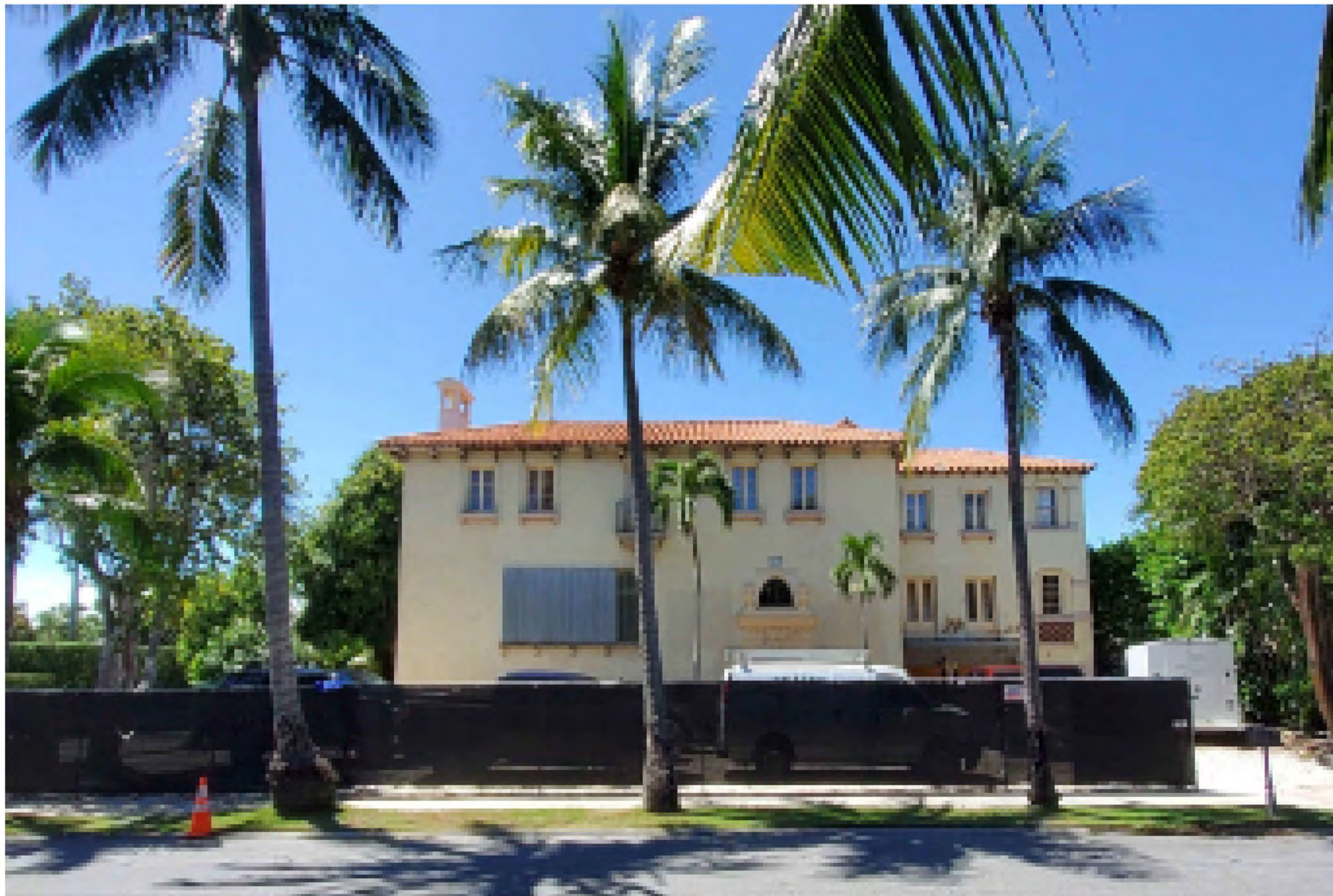
SUBJECT PROPERTY: EAST ELEVATION (front)
