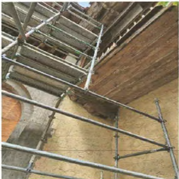
PHOTO 4 - West Balcony – Looking at underside of balcony floor with end outrigger
