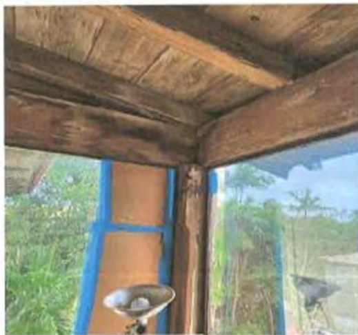
PHOTO 6 - West Balcony – Looking at southwest corner of roof framing
