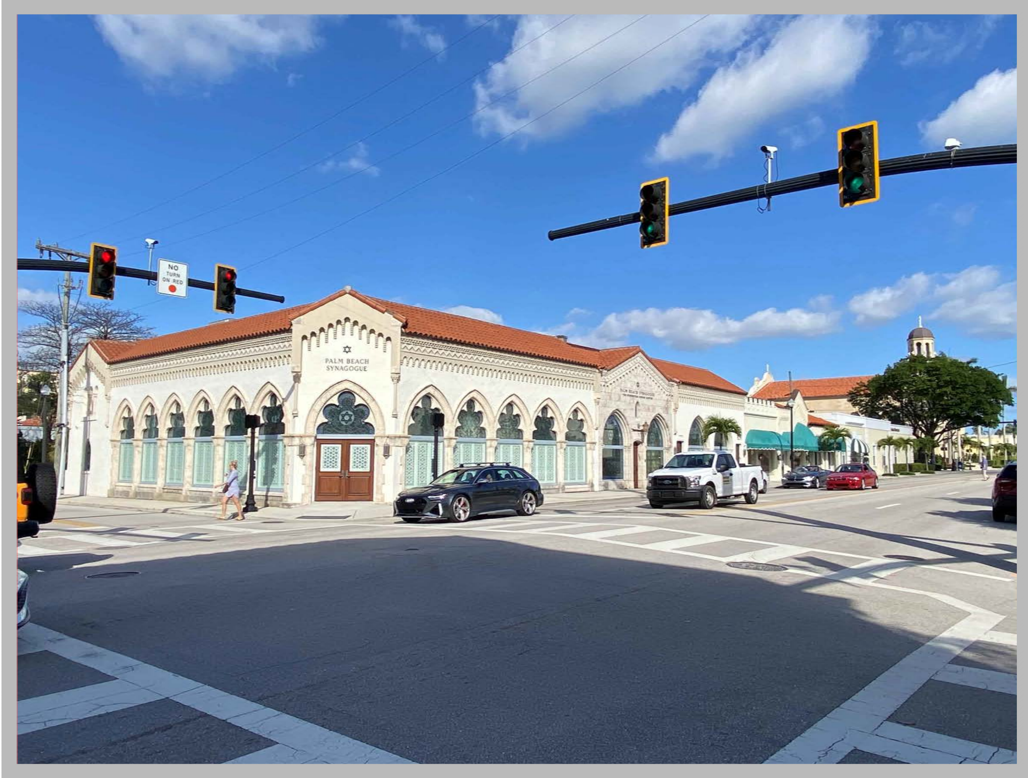
North-West Corner looking North-West
