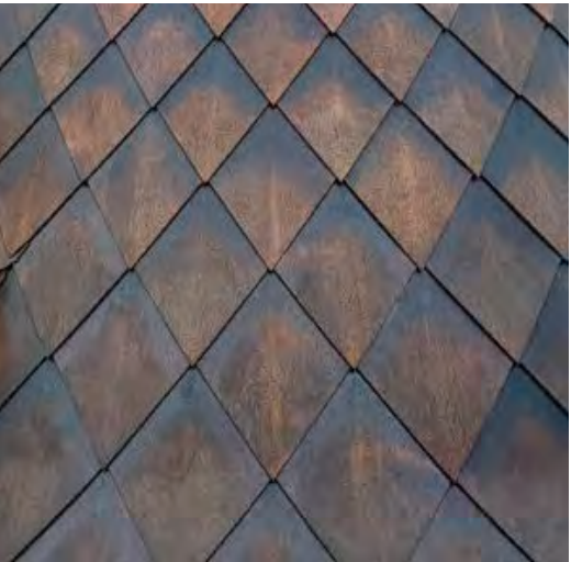
GUEST HOUSE: CUSTOM METAL ROOF, DIAMOND PATTERN: COPPER
