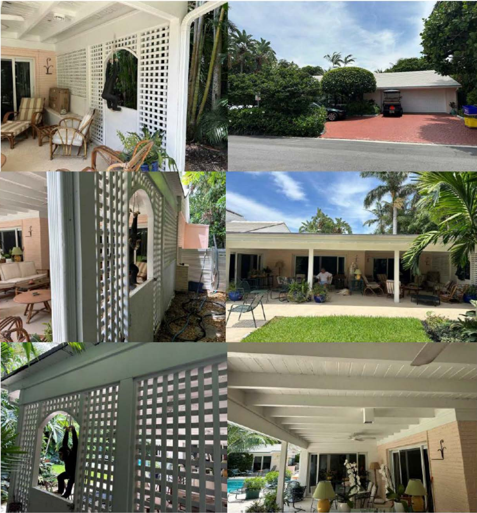
EXISTING TERRACE TO BE REPAIRED
