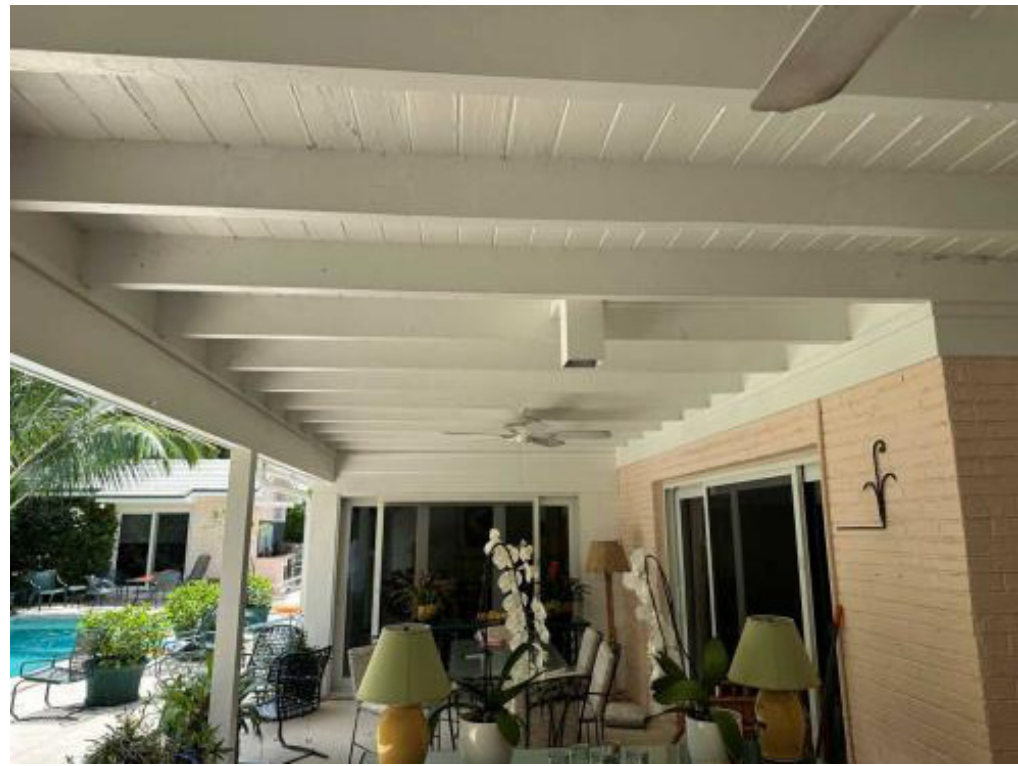
UNDER TERRACE (WEST)
