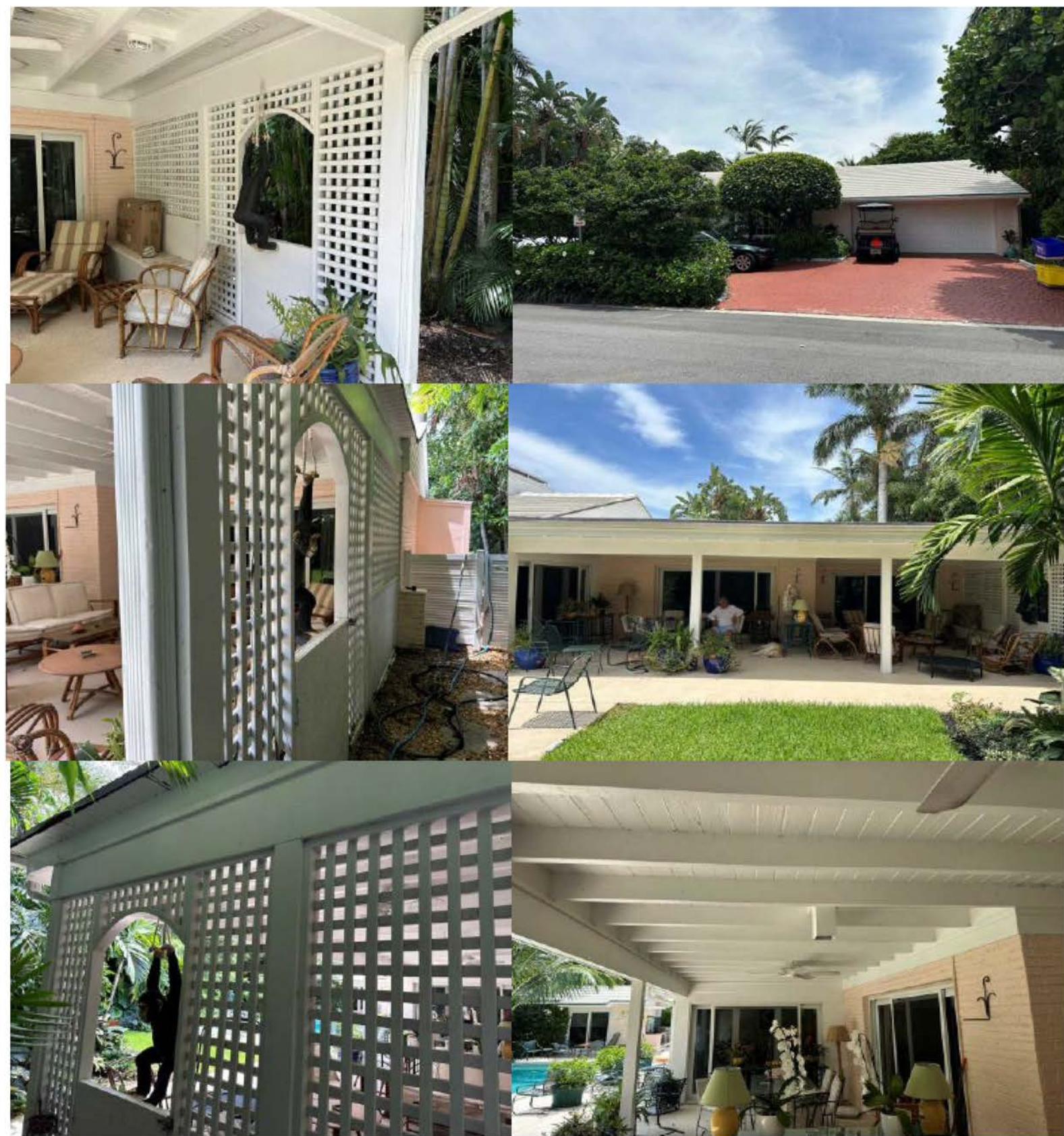
EXISTING TERRACE TO BE REPAIRED
