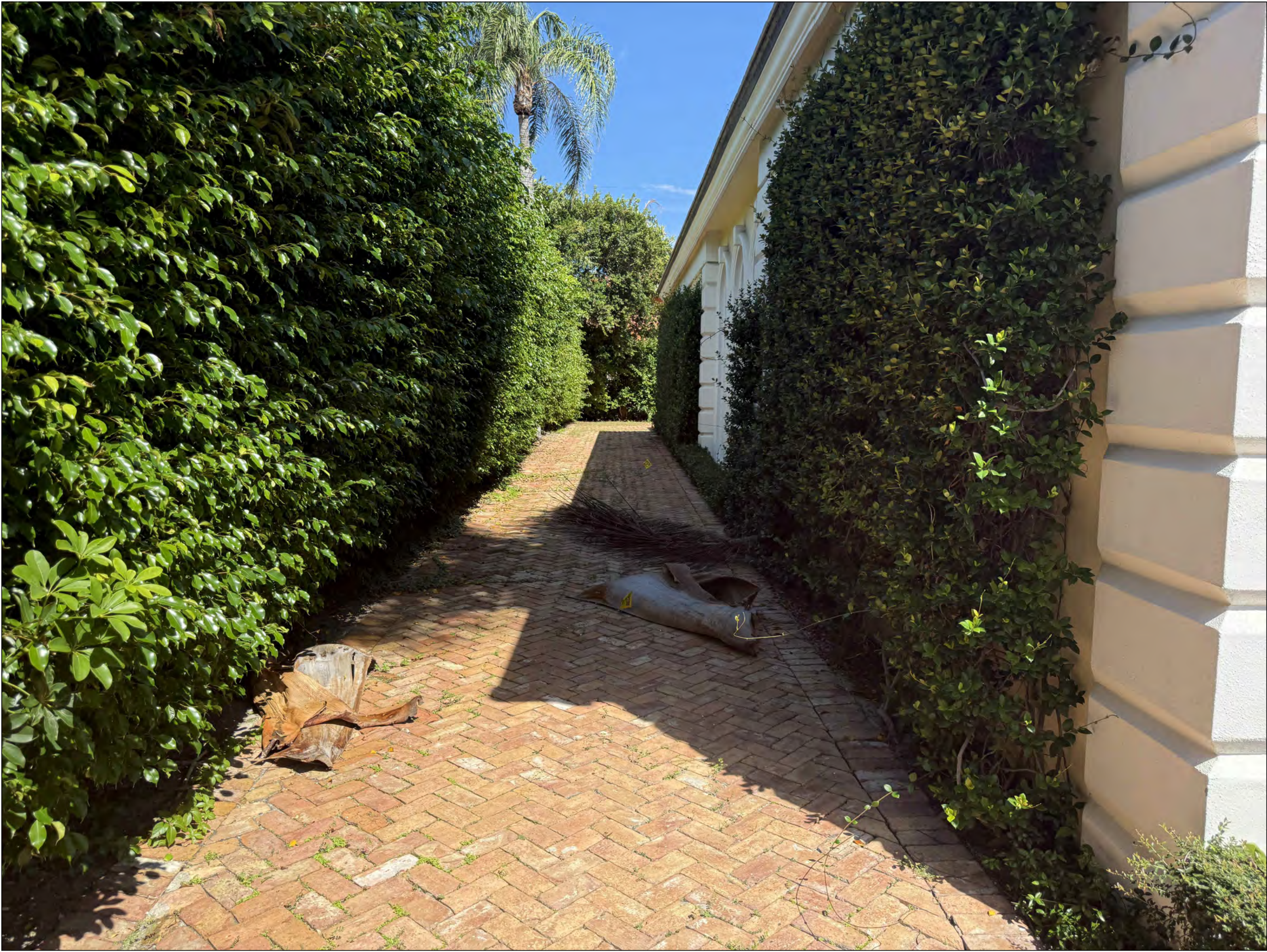
EXISTING DRIVEWAY LOOKING NORTH
