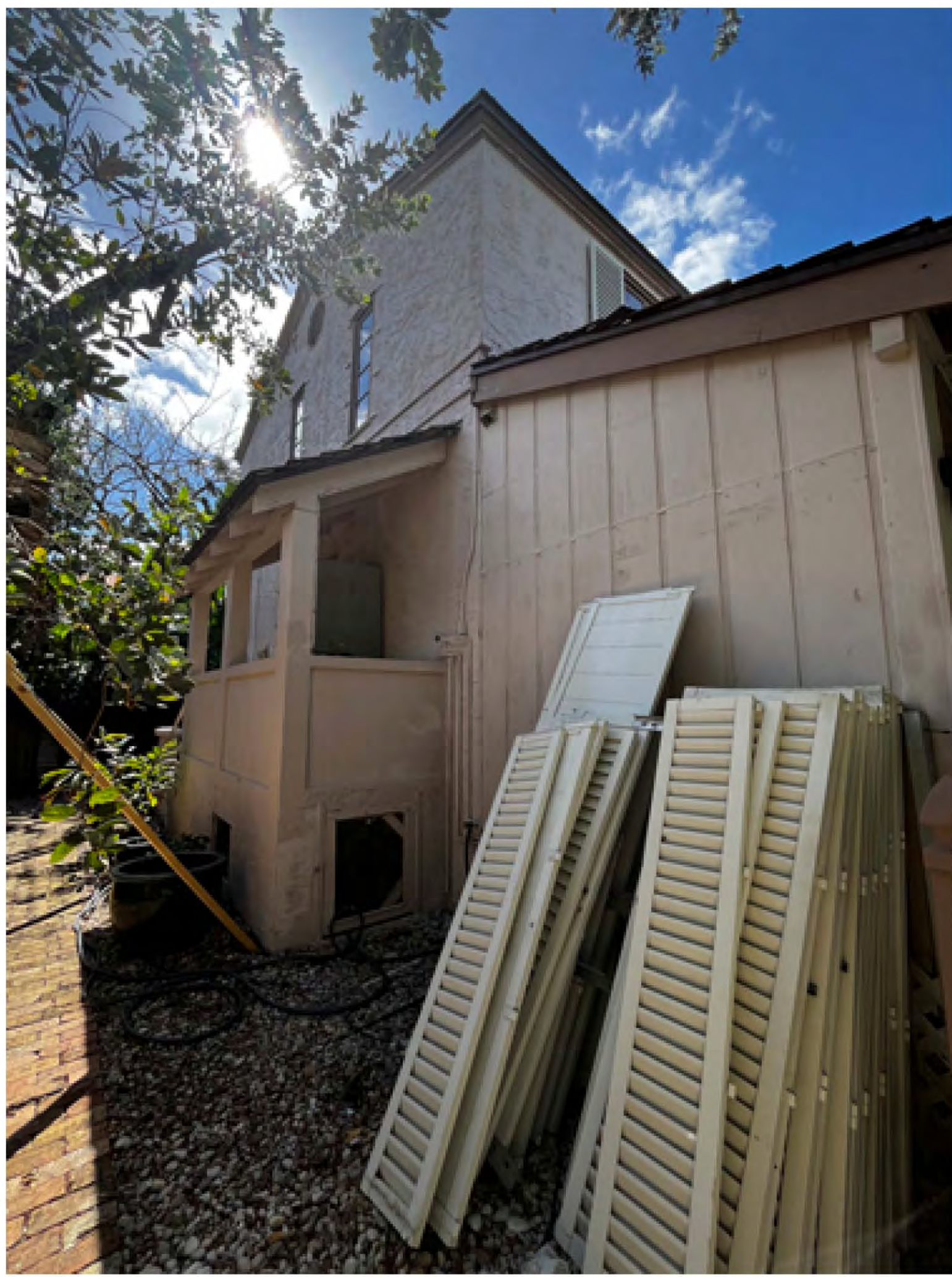
4/SP2 WEST SIDE OF NORTH ELEVATION
