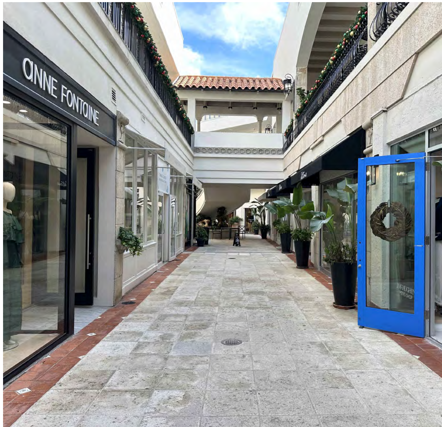
View to East Courtyard
