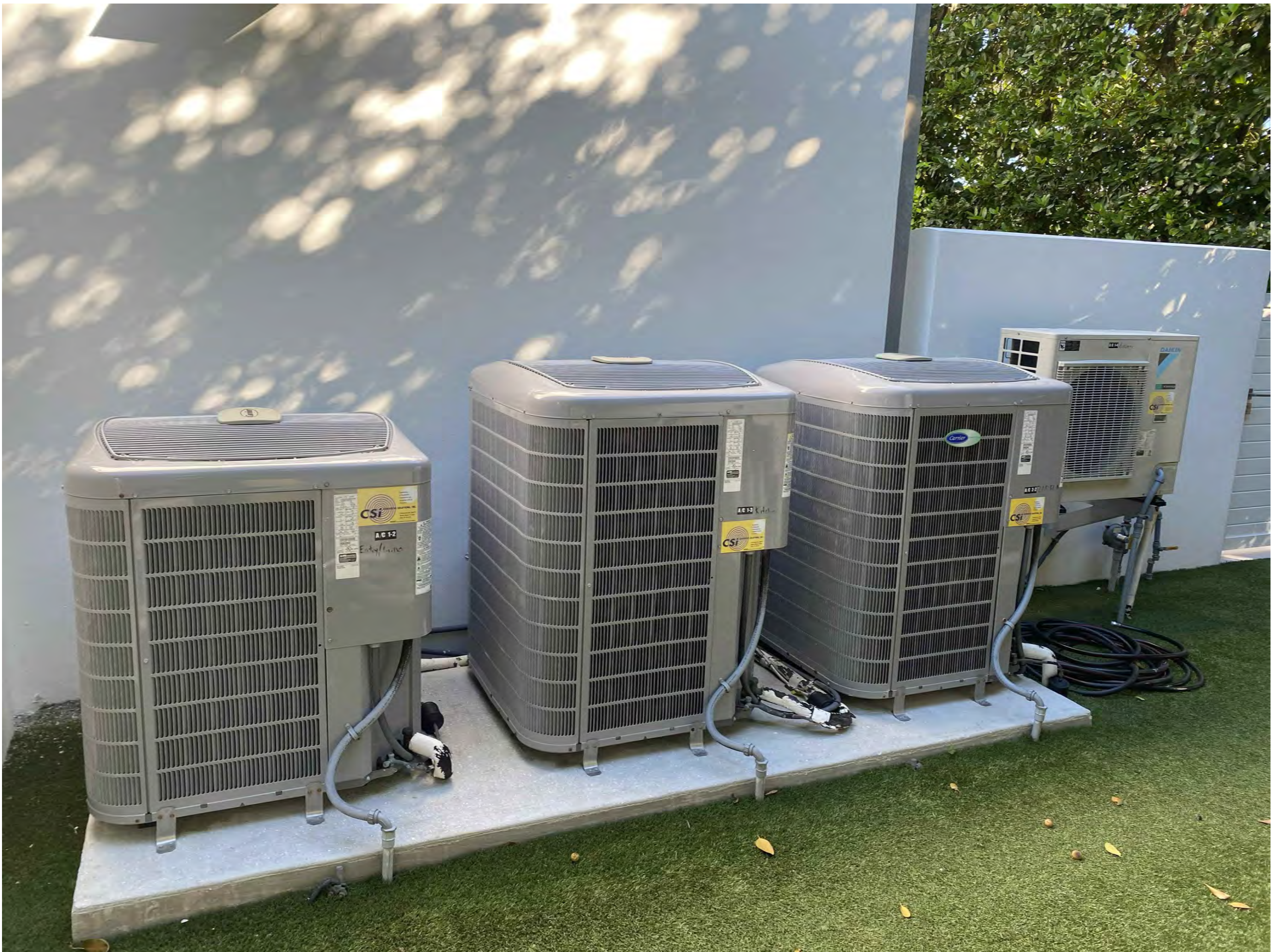
WEST EQUIPMENT AREA
