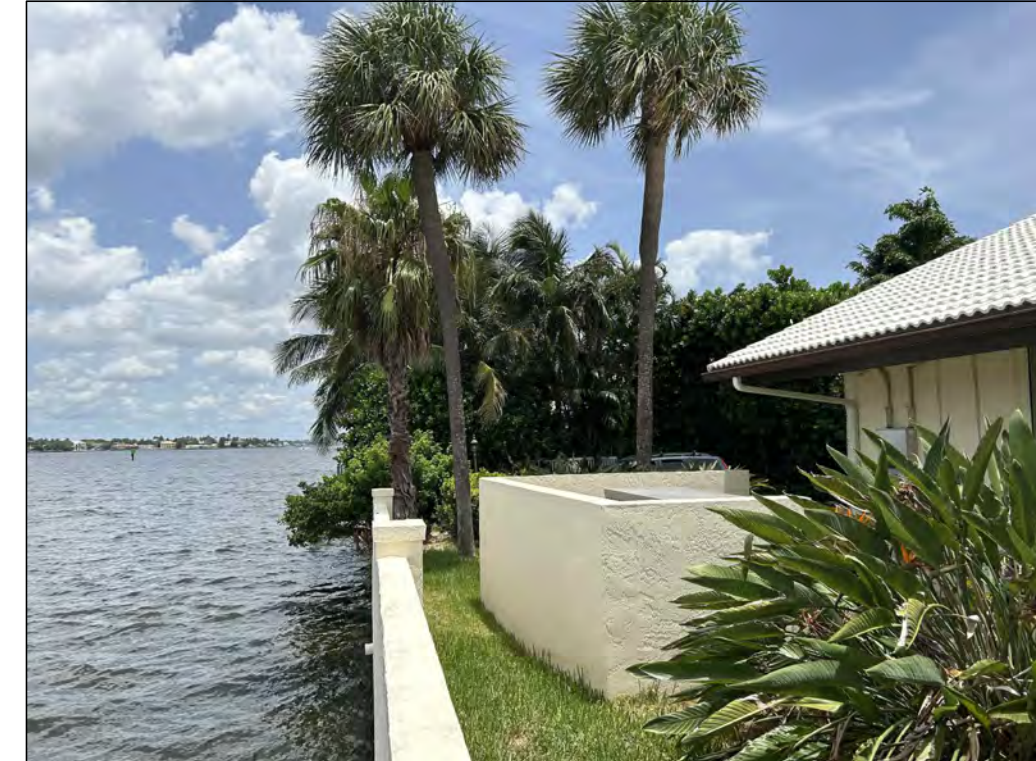
5 GENERATOR SCREEN WALL AREA
