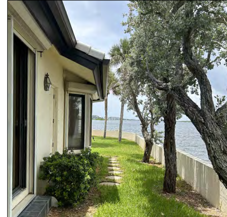
7 SIDE WALKWAY TO REAR
