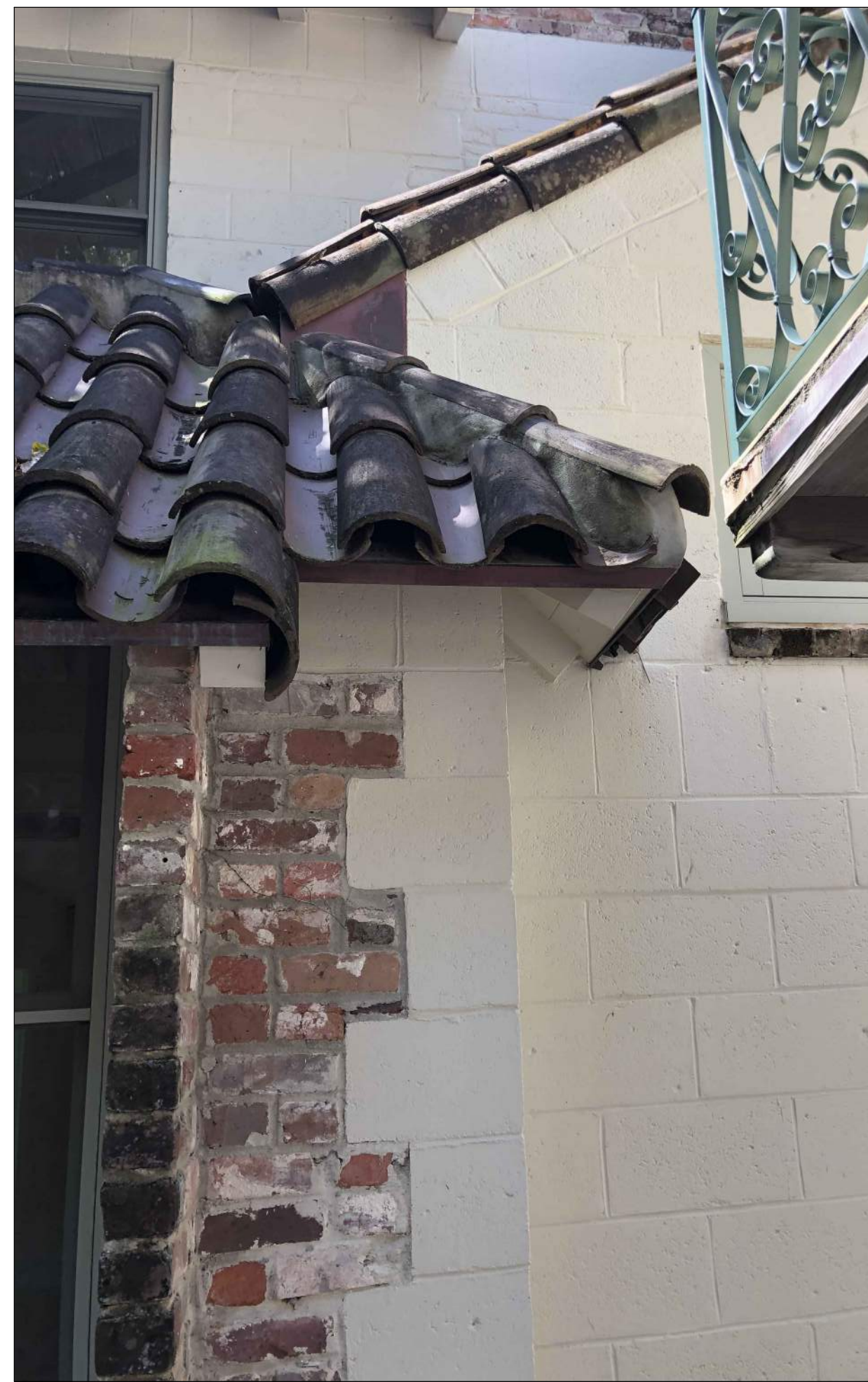
2 INTERNAL ENTRY FACADE
