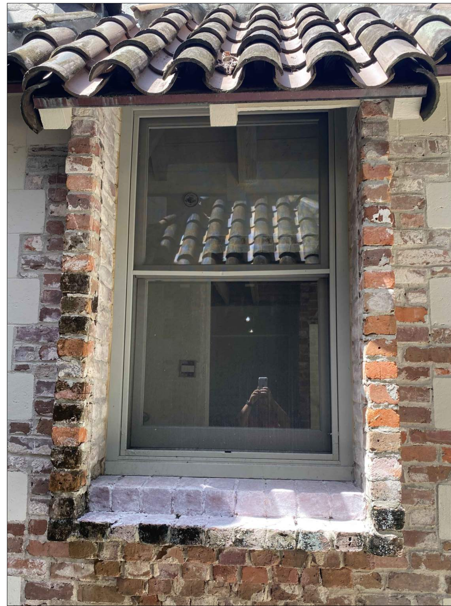
3 INTERNAL ENTRY FACADE
