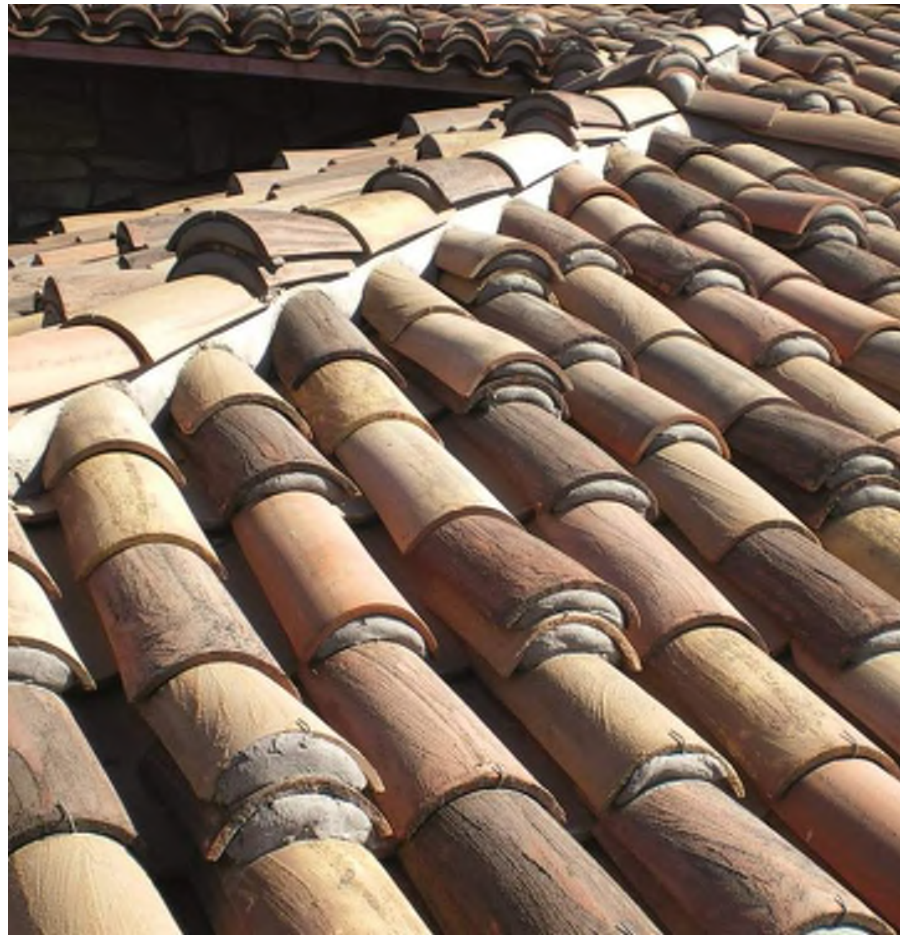
TAPERED MISSION BARREL TILE COLOR: MATCH EXISTING. SUBTLE MORTAR WEEPS
