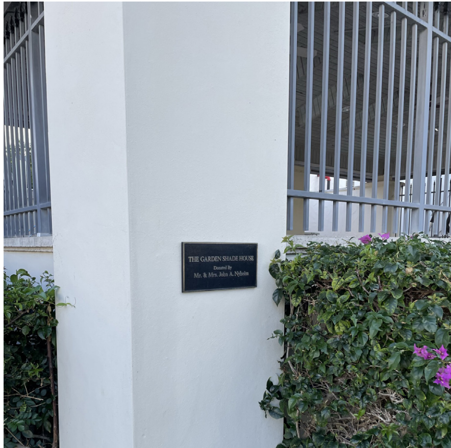
STUCCO, ORNAMENTAL FENCING/GATE
