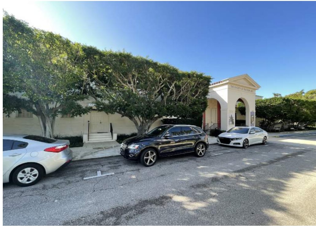
EXISTING PHOTOS - NORTH ELEVATION
