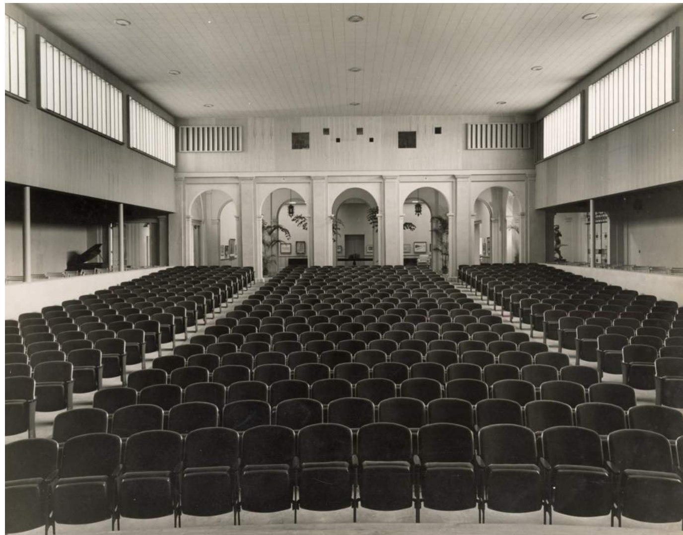
5 PHOTO - AUDITORIUM LOOKING EAST TO FORMER LOGGIA, CIRCA 1947 B-1.0.1 NTS - COURTESY HISTORICAL SOCIETY OF PALM BEACH COUNTY
