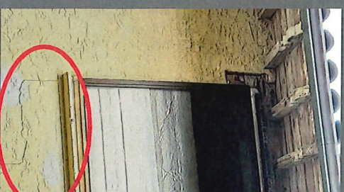
DIAGONAL CRACK IN THE TERRACOTTA WALL UNDER WINDOW SILL LOOKING FROM OUTSIDE
