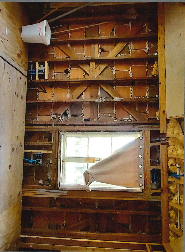
BROKEN TERRACOTTA TILES MIXED WITH CMU AND BRICK INFILL AT DIFFERENT LOCATION
