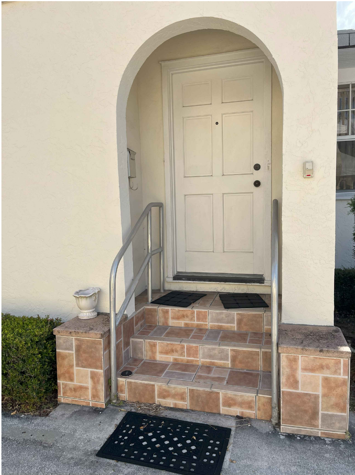
1 EXISTING FRONT ENTRANCE VIEWPORT 1
