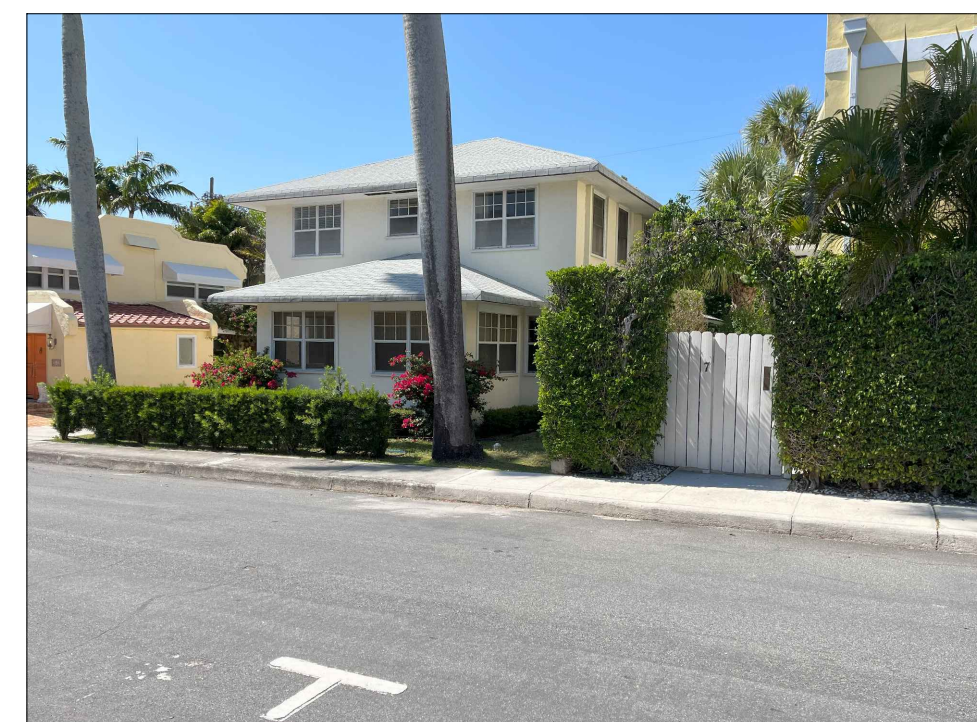
SUBJECT PROPERTY 211 PARK AVENUE
