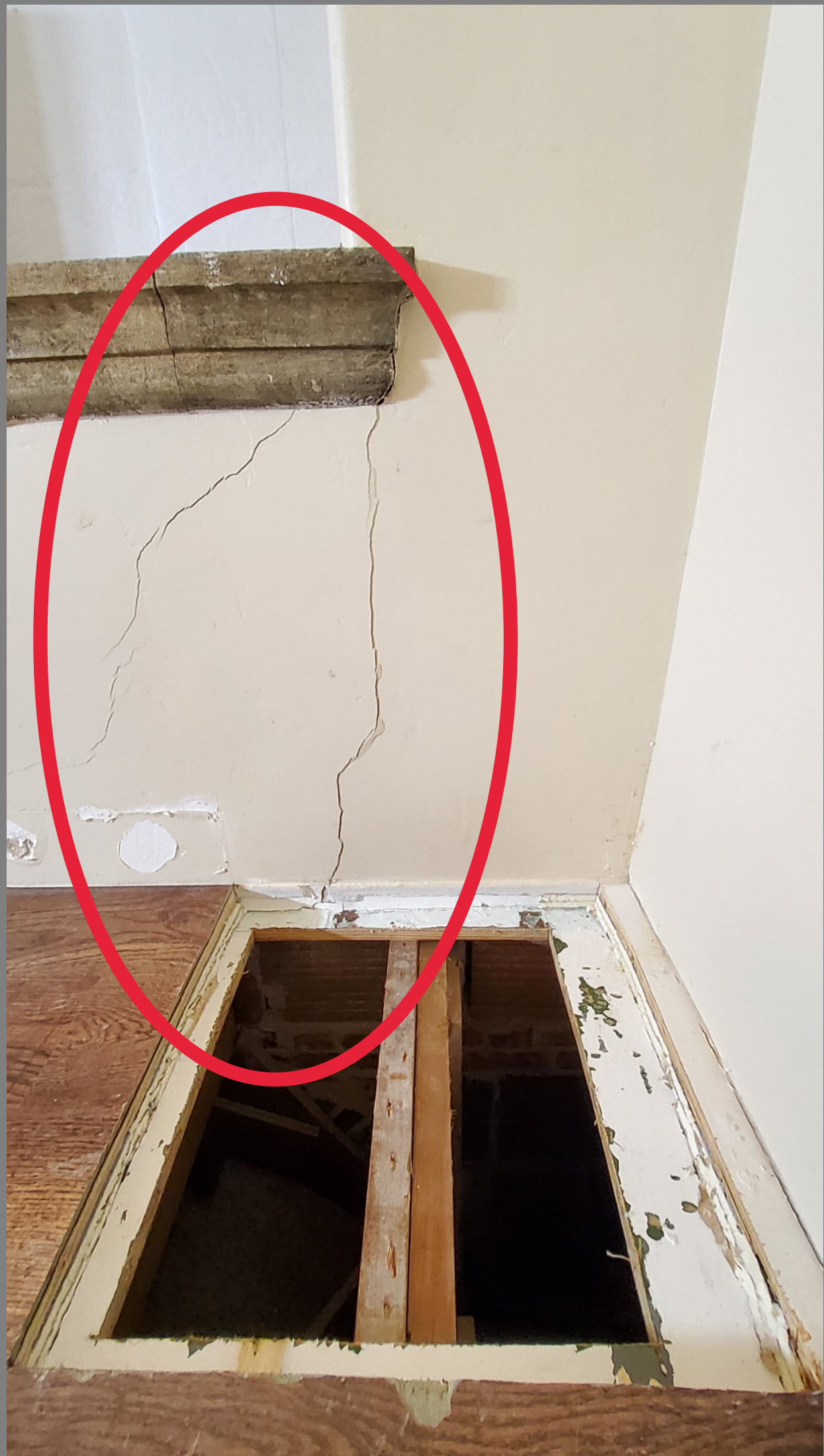
DIAGONAL CRACK IN THE TERRACOTTA WALL BELOW WINDOW SILL LOOKING FROM INSIDE
