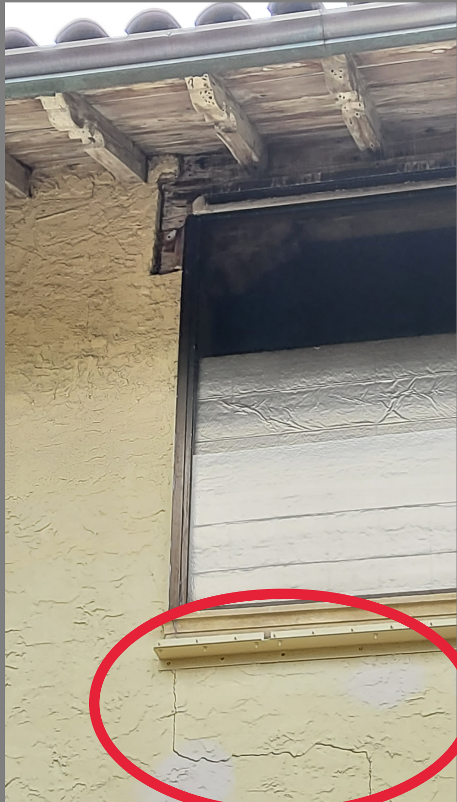
DIAGONAL CRACK IN THE TERRACOTTA WALL UNDER WINDOW SILL LOOKING FROM OUTSIDE
