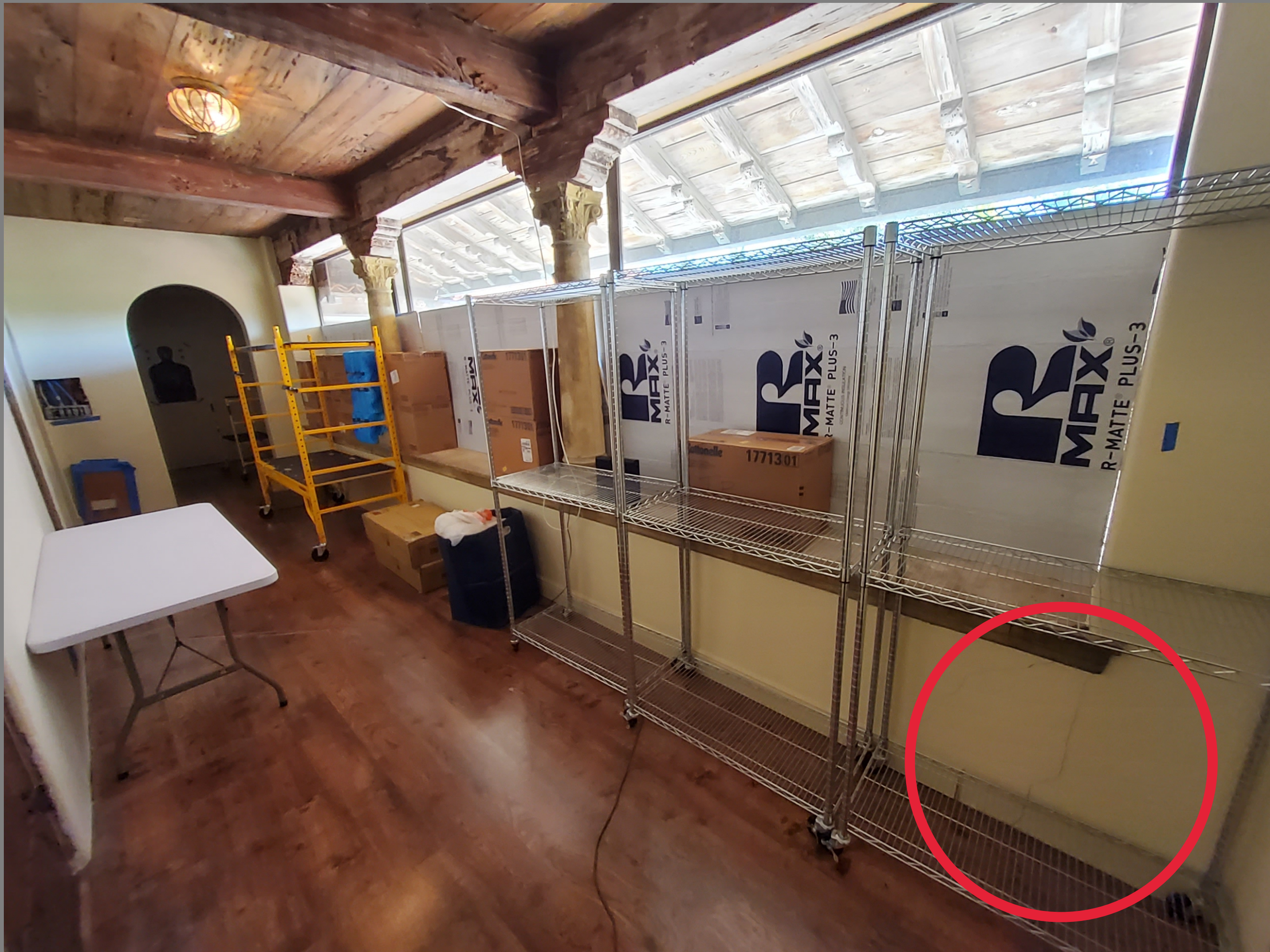
DIAGONAL CRACK IN THE TERRACOTTA WALL BELOW WINDOW SILL LOOKING FROM INSIDE
