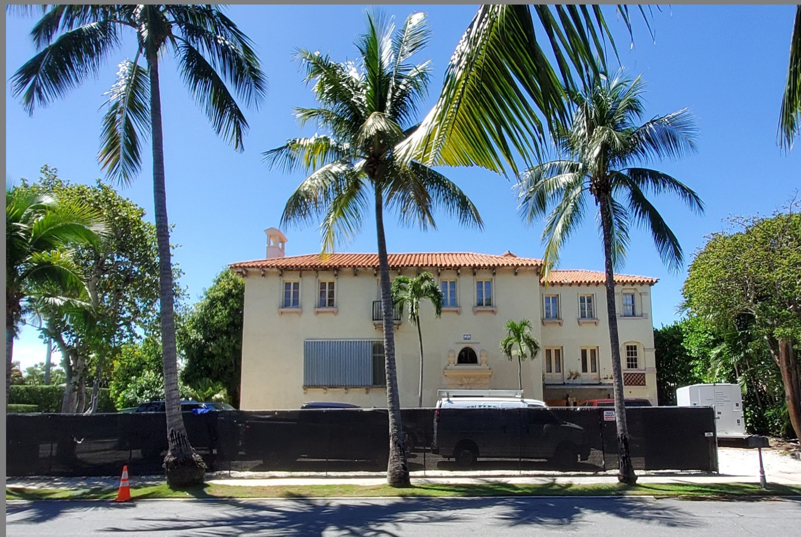
SUBJECT PROPERTY: EAST ELEVATION (front)
