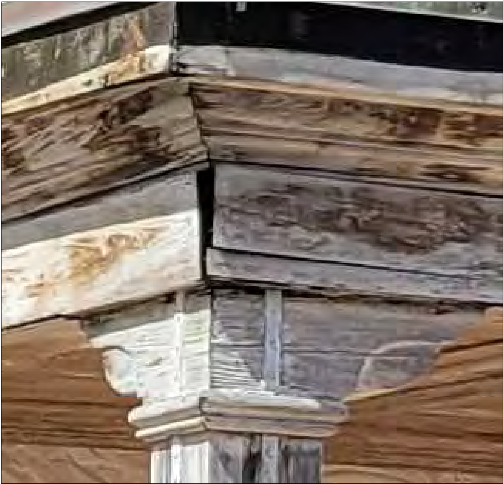
3 WOOD BEAMS, COLUMNS, AND DETAILS CYPRESS TO MATCH ORIGINAL
