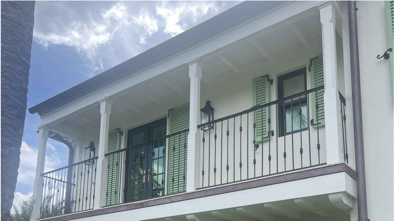
02 ————— EXISTING FRONT RAILING
