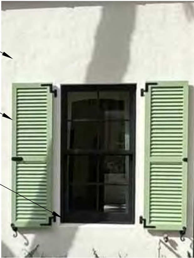
Windows and shutters
