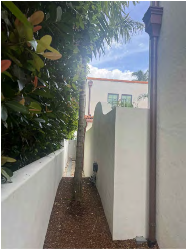
Low wall located at the west side of the property
