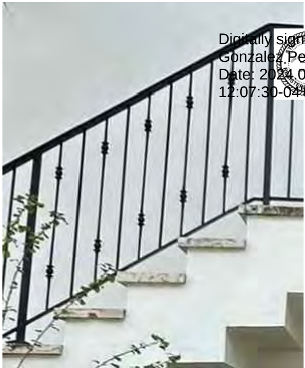
02 EXISTING RAILING PHOTO
