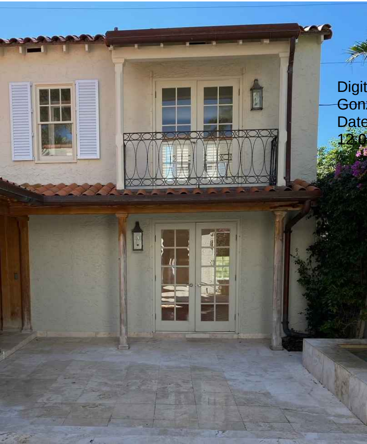
03 ————— EXISTING COURTYARD RAILING IN 2020
