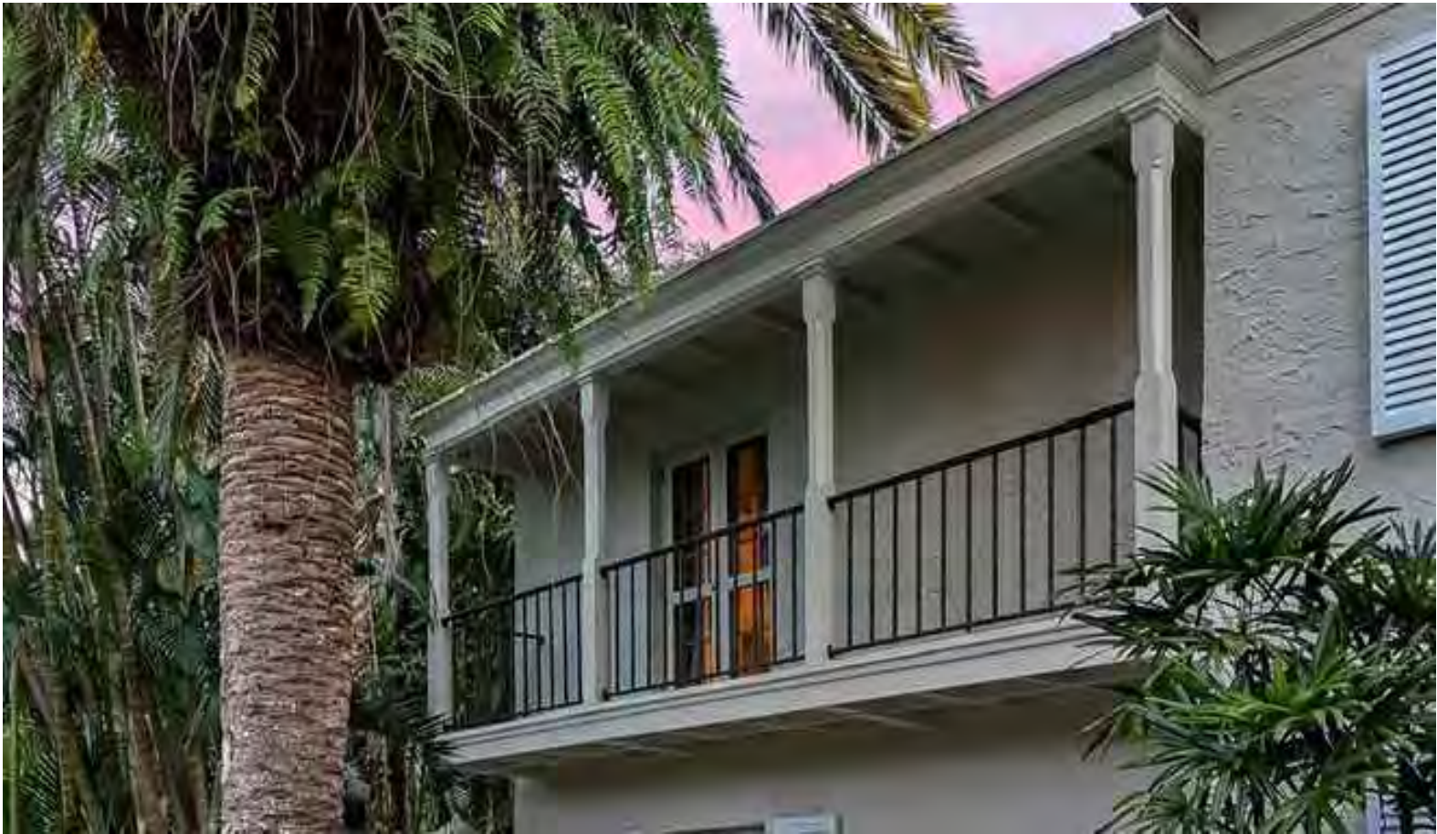
01 ————— EXISTING RAILING IN 2020
