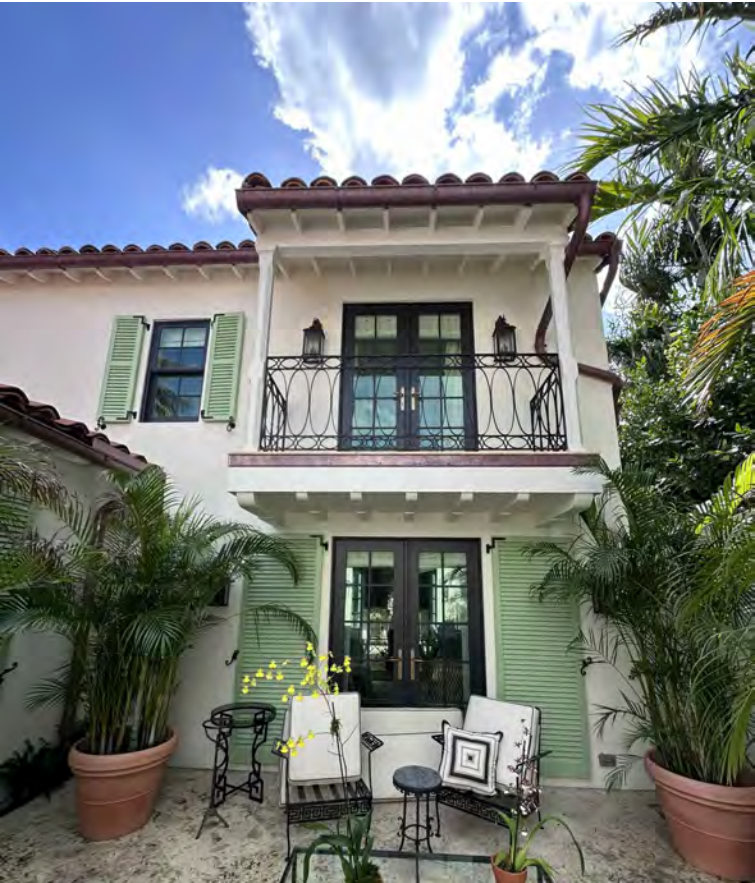
04 ————— EXISTING COURTYARD RAILING
