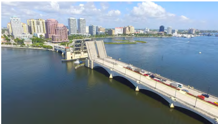
Figure 7 Royal Park Bridge Opening
