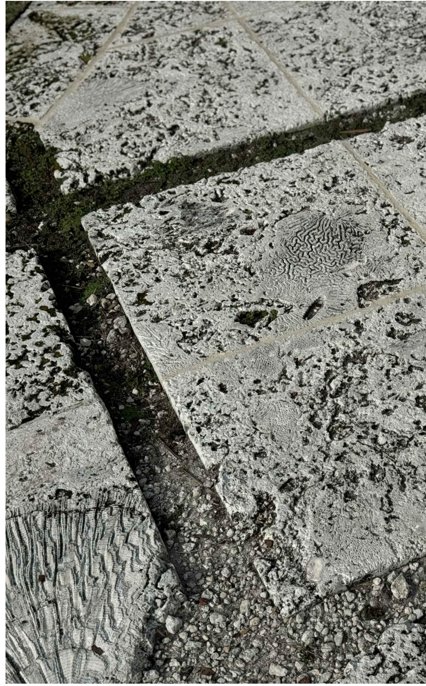
C. EXAMPLE OF PAVING DAMAGE AT FRONT PARKING COURT
