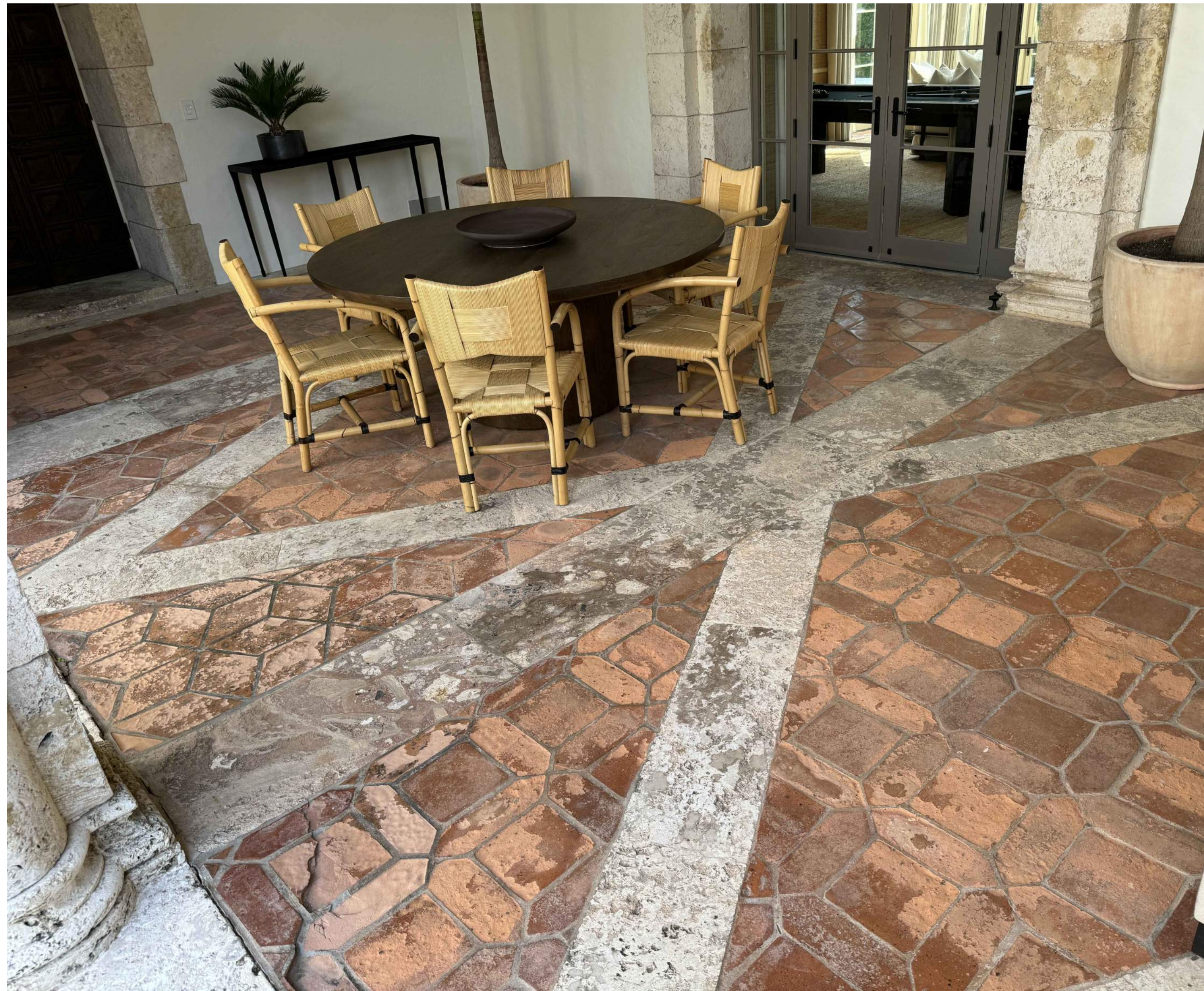
G. EXAMPLE OF TILE DAMAGE AT LOGGIA
