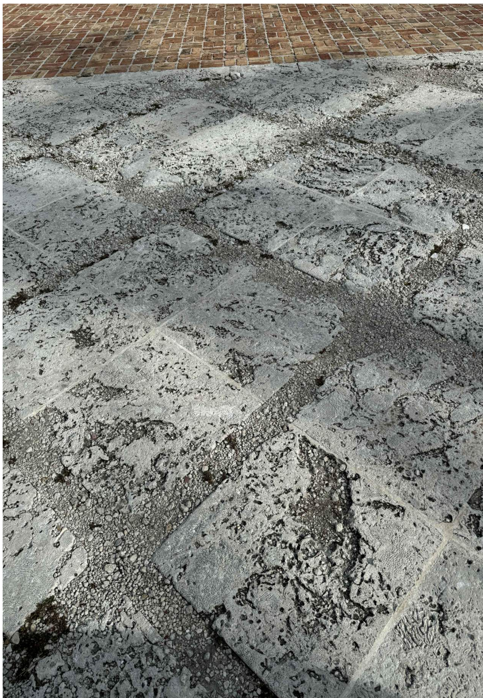
B. EXAMPLE OF PAVING DAMAGE AT FRONT PARKING COURT
