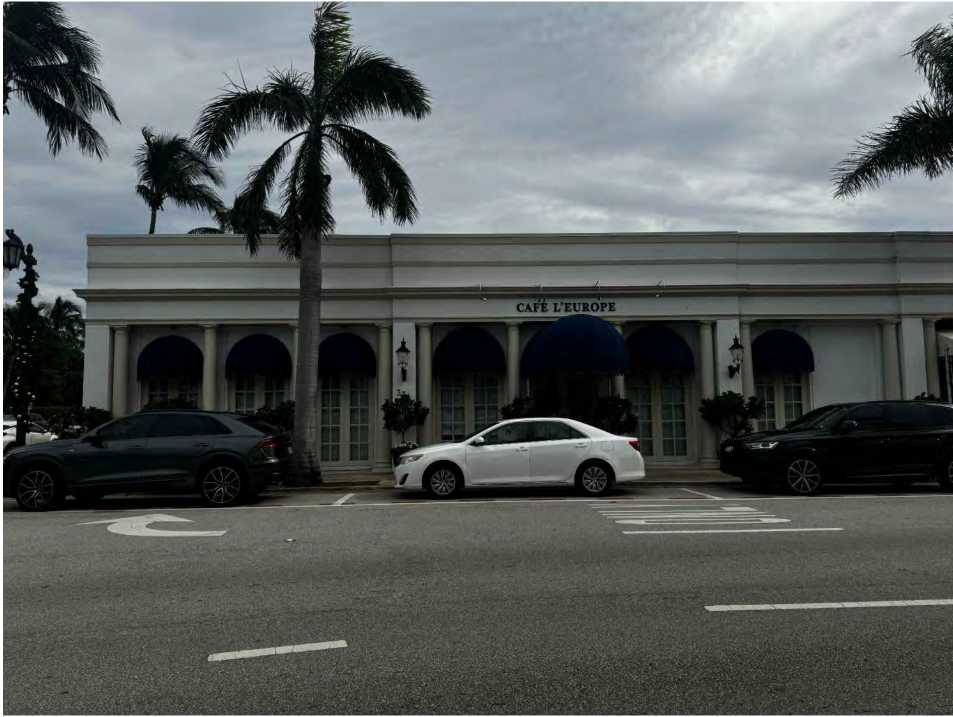
331 S COUNTY RD
