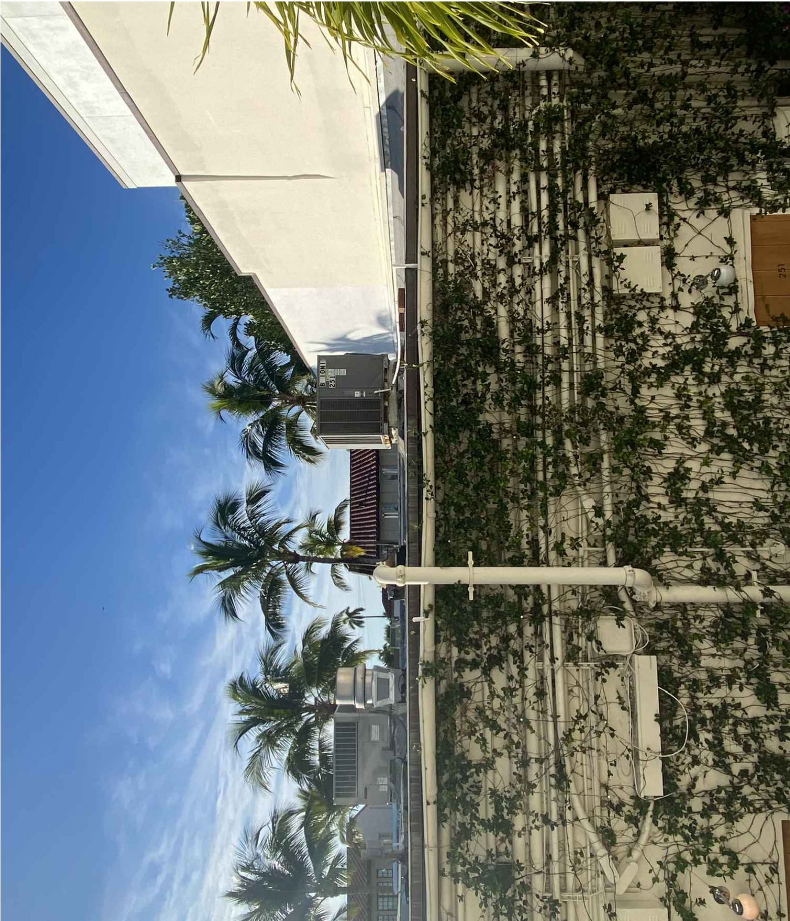
Existing Rooftop Vines
