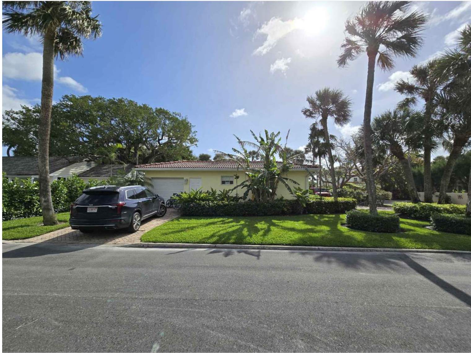
B: WESTERN SIDE WITH GARAGE
