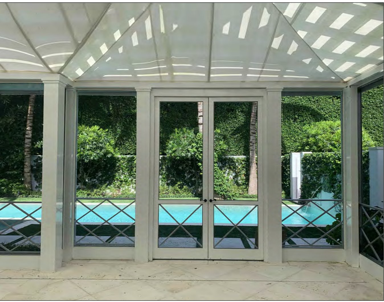
Ⓓ PERGOLA FROM INSIDE
