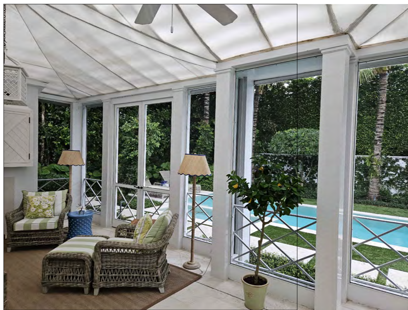
Ⓓ PERGOLA - INTERIOR LOOKING EAST
