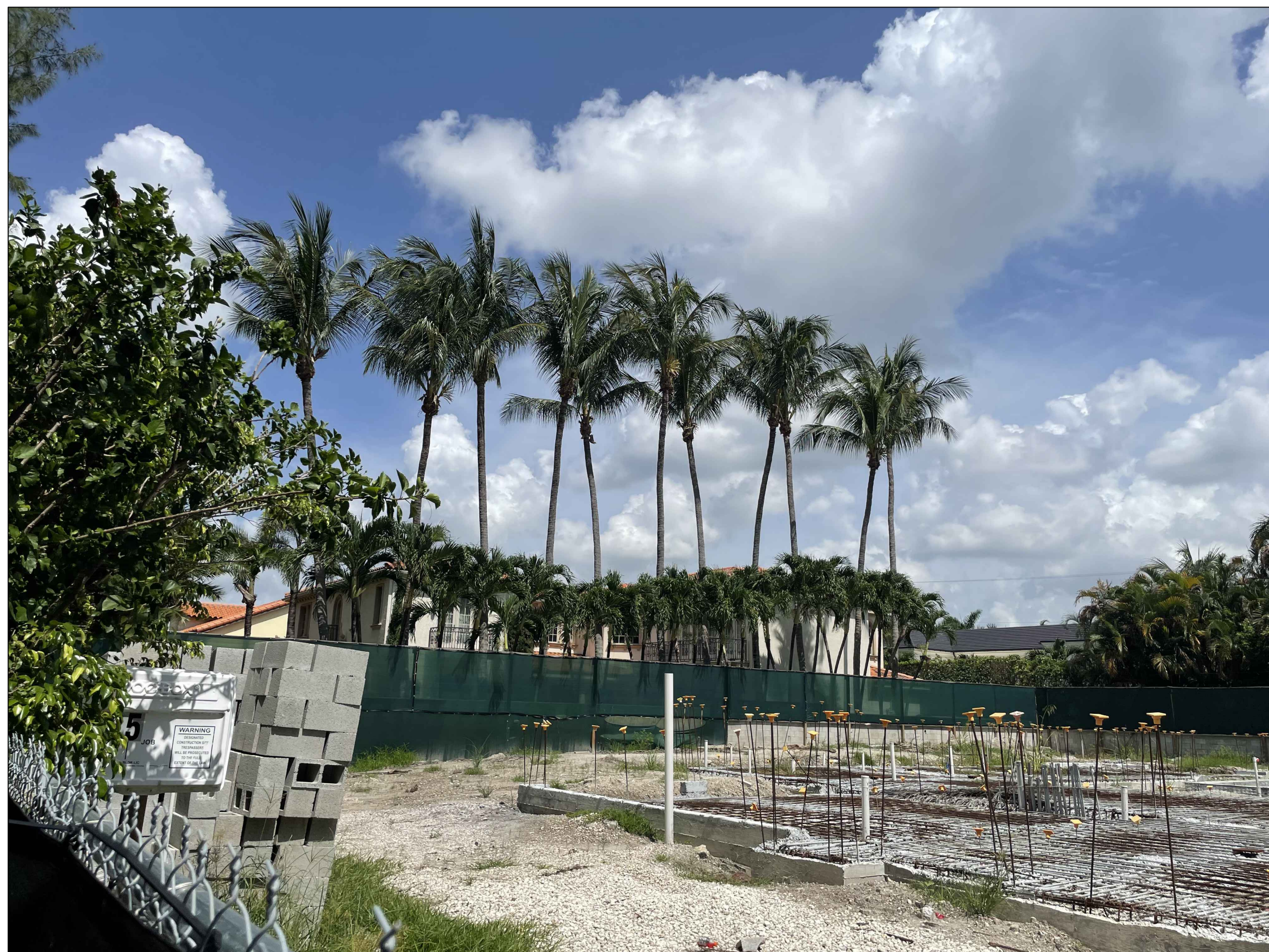
EXISTING SITE FACING WEST
