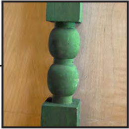
GREEN WOODEN RAILINGS TO MATCH HISTORIC SAMPLE
