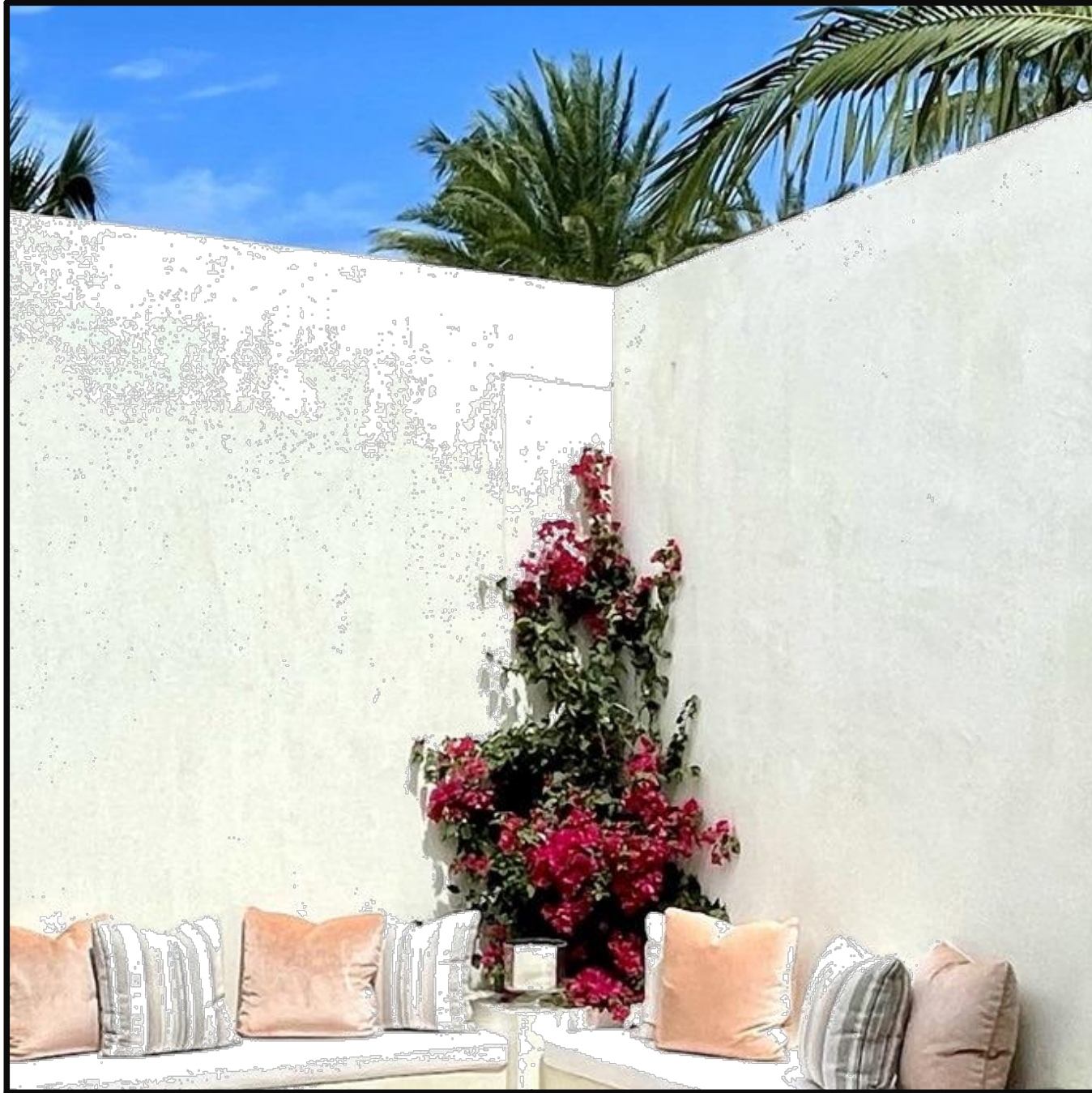
EXTERIOR MASONRY WALL FINISH: STUCCO "HAND OF THE CRAFTSMAN" W/ PAINTED LIME WASH FINISH.
