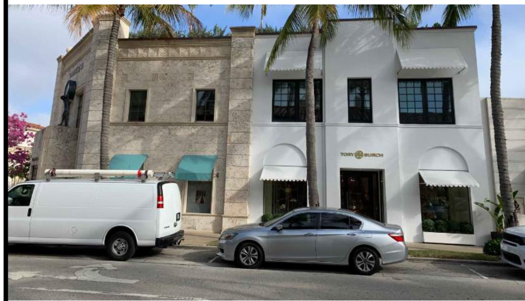
259 WORTH - 3 STORY NORTH SIDE WORTH AVENUE
