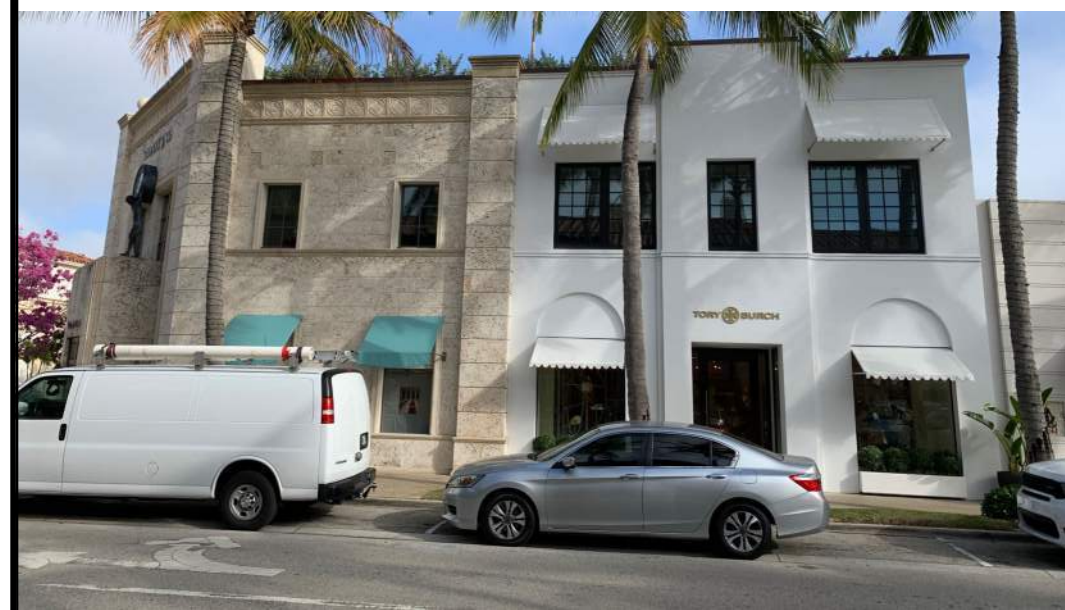
259 WORTH - 3 STORY NORTH SIDE WORTH AVENUE
