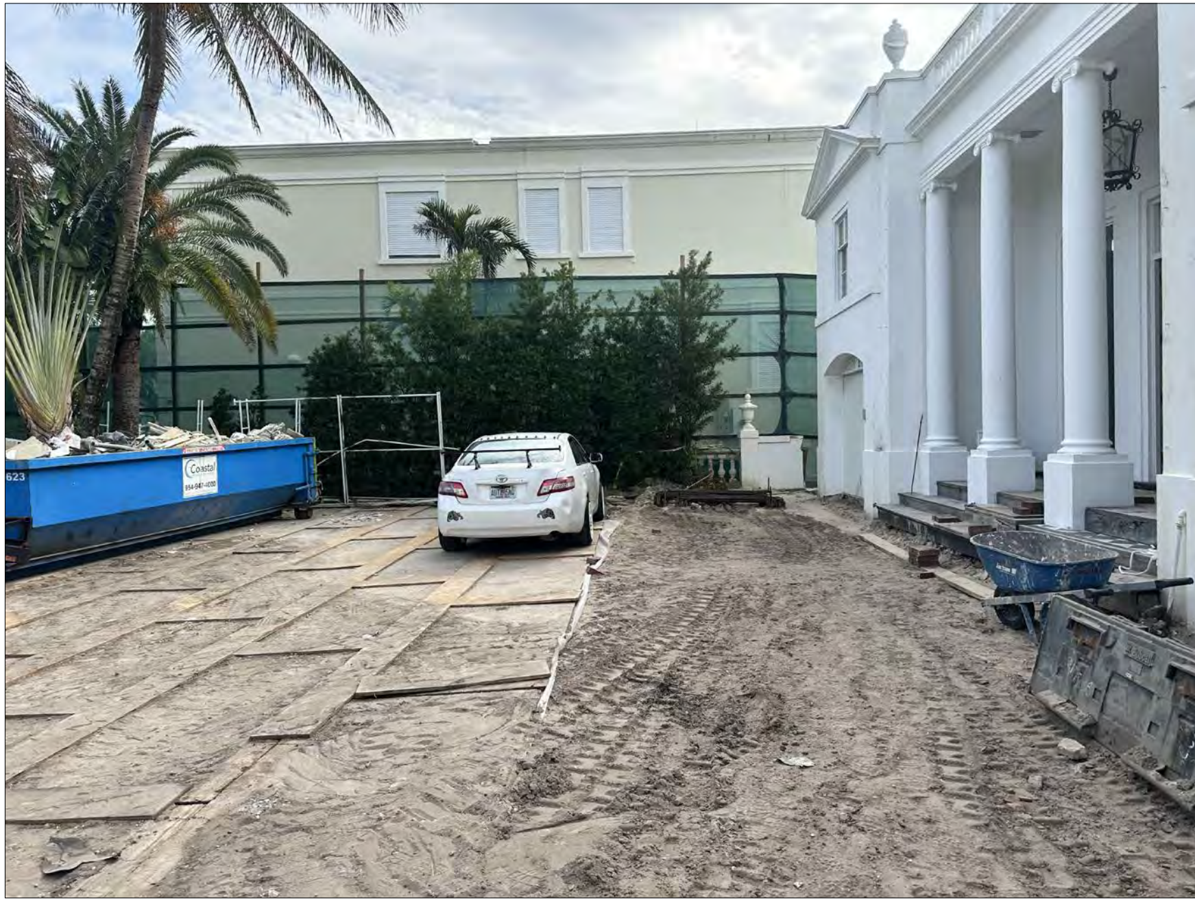
PHOTO 1: DRIVE WAY AREA
