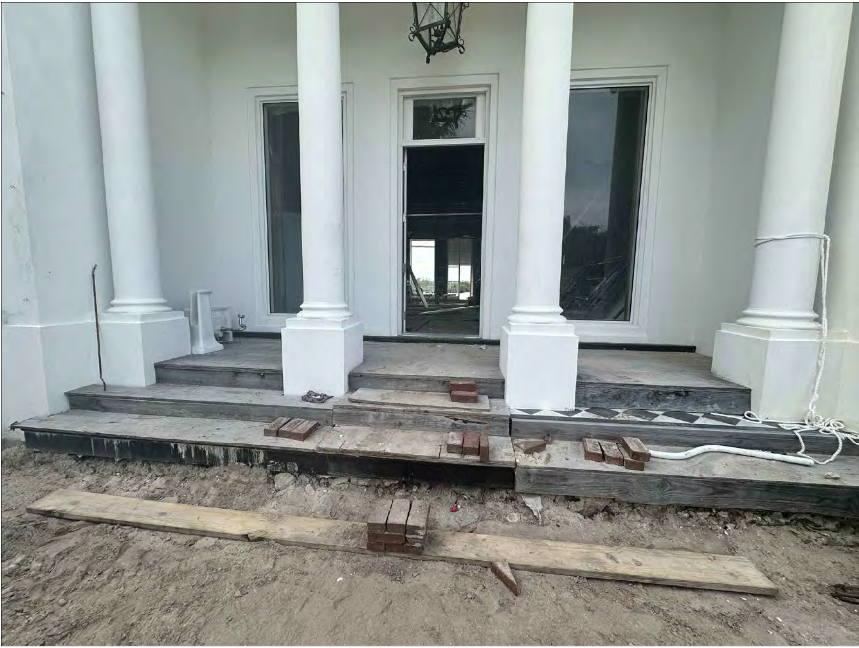
PHOTO 3: FRONT ENTRY WAY
