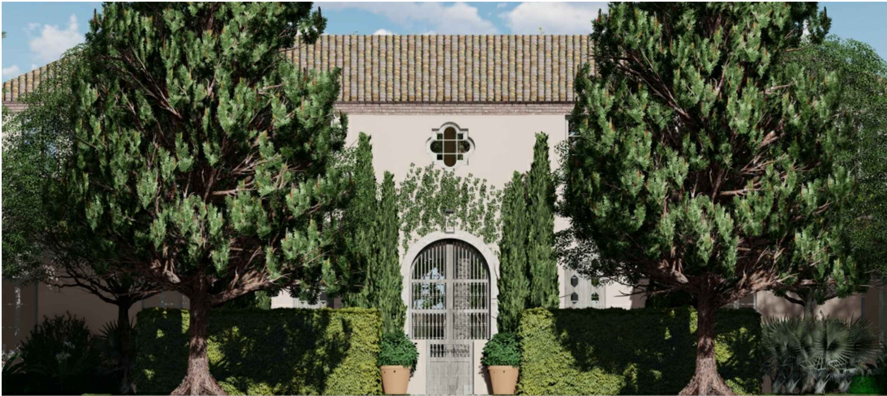
225 WELLS ROAD PALM BEACH FLORIDA
