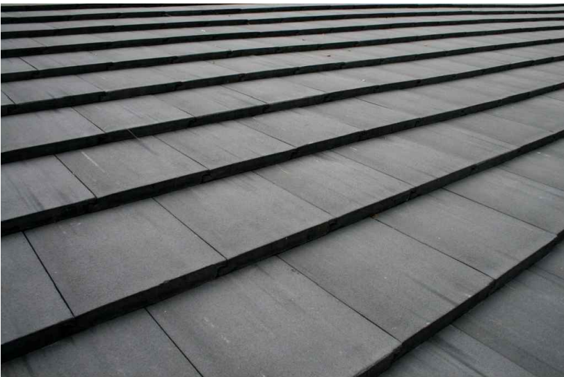
FLAT CEMENT TILE SLOPED ROOFS
