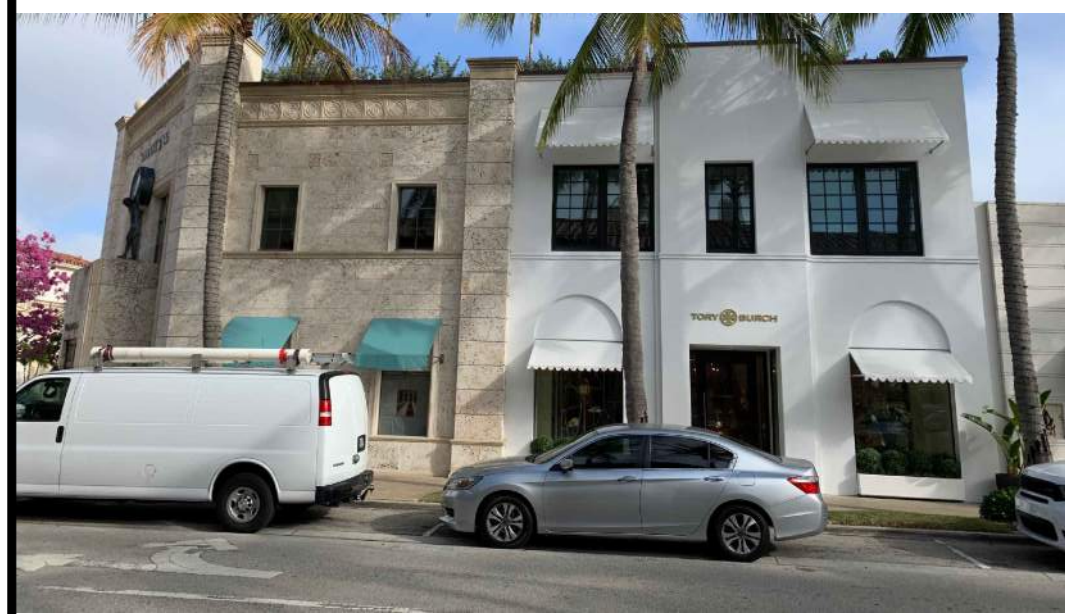
259 WORTH - 3 STORY NORTH SIDE WORTH AVENUE
