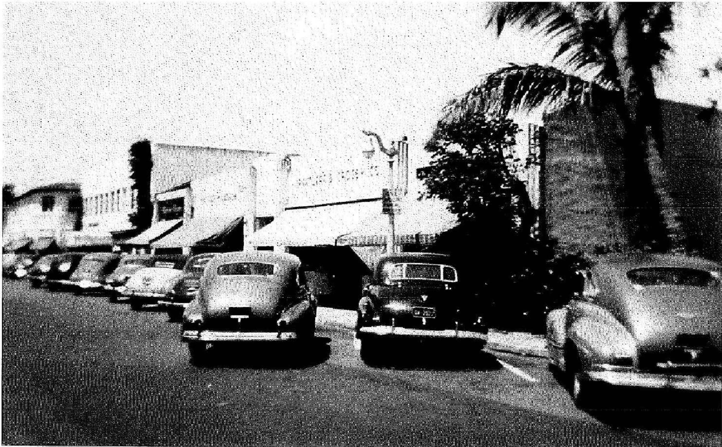
1948 VIEW FROM EAST 251-245 WORTH AVENUE
