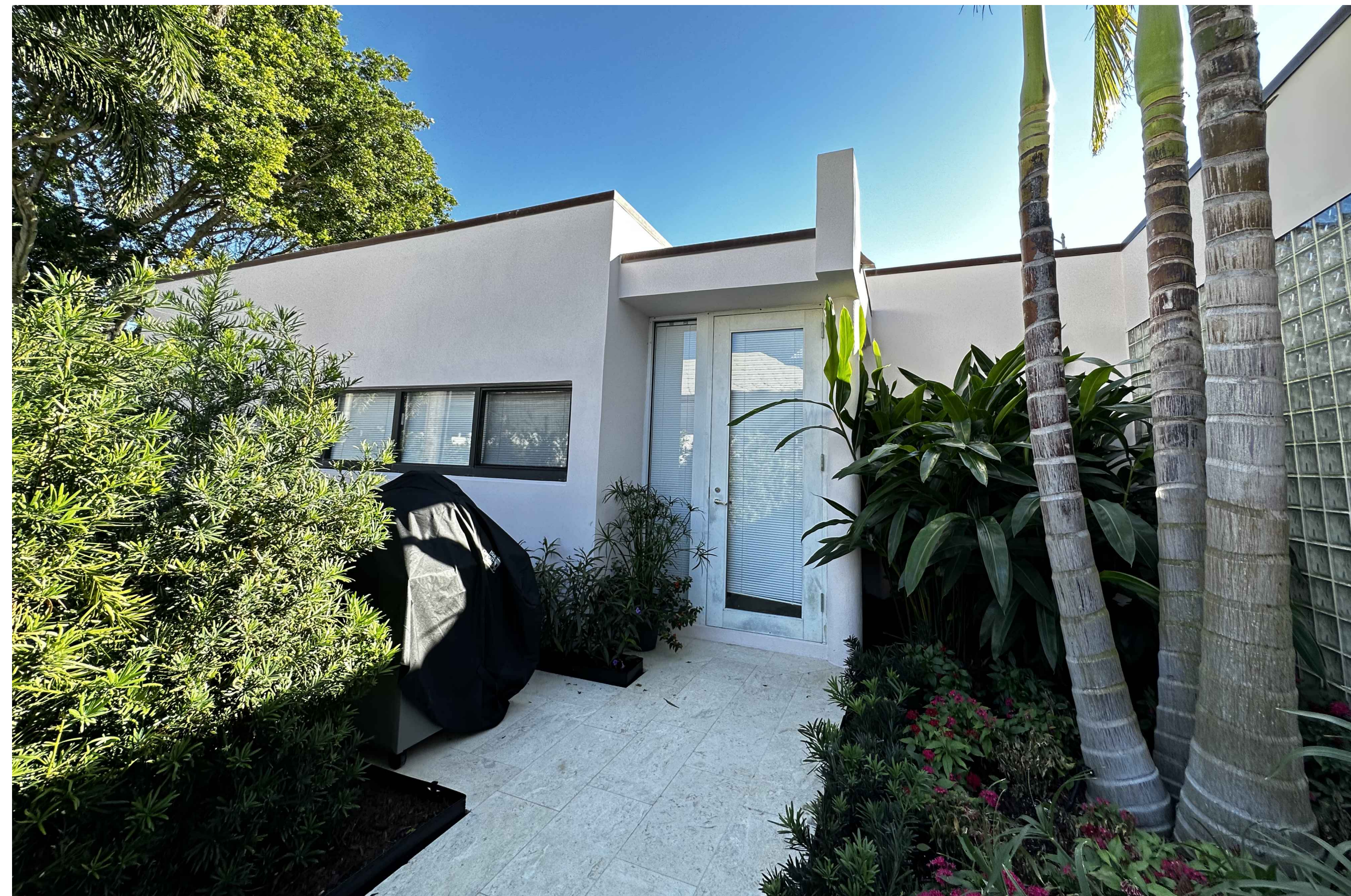
288 Sandpiper Drive West Elevation Subject Property
