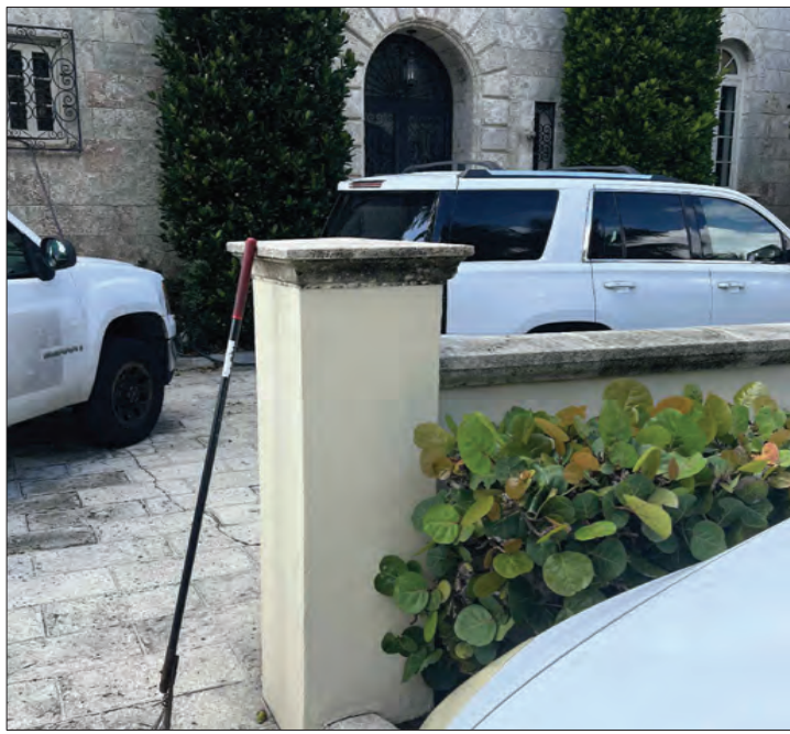
Photograph of existing wall and column, above. Column and wall cap are to be removed. Wall to be extended over footprint of existing column. New wall cap to be 4" thick FL Coral, to match Fatio wall cap at house shown below.
