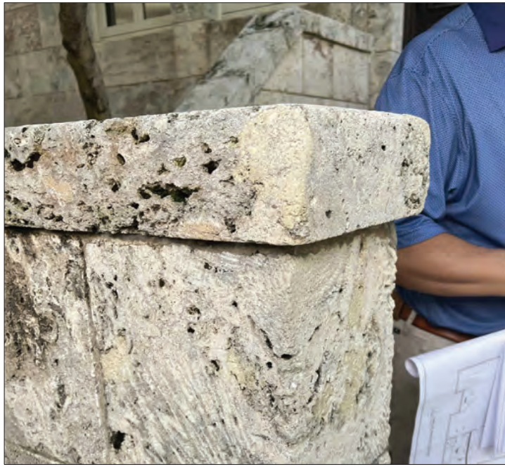
Photograph of existing wall and column, above. Column and wall cap are to be removed. Wall to be extended over footprint of existing column. New wall cap to be 4" thick FL Coral, to match Fatio wall cap at house shown below.
