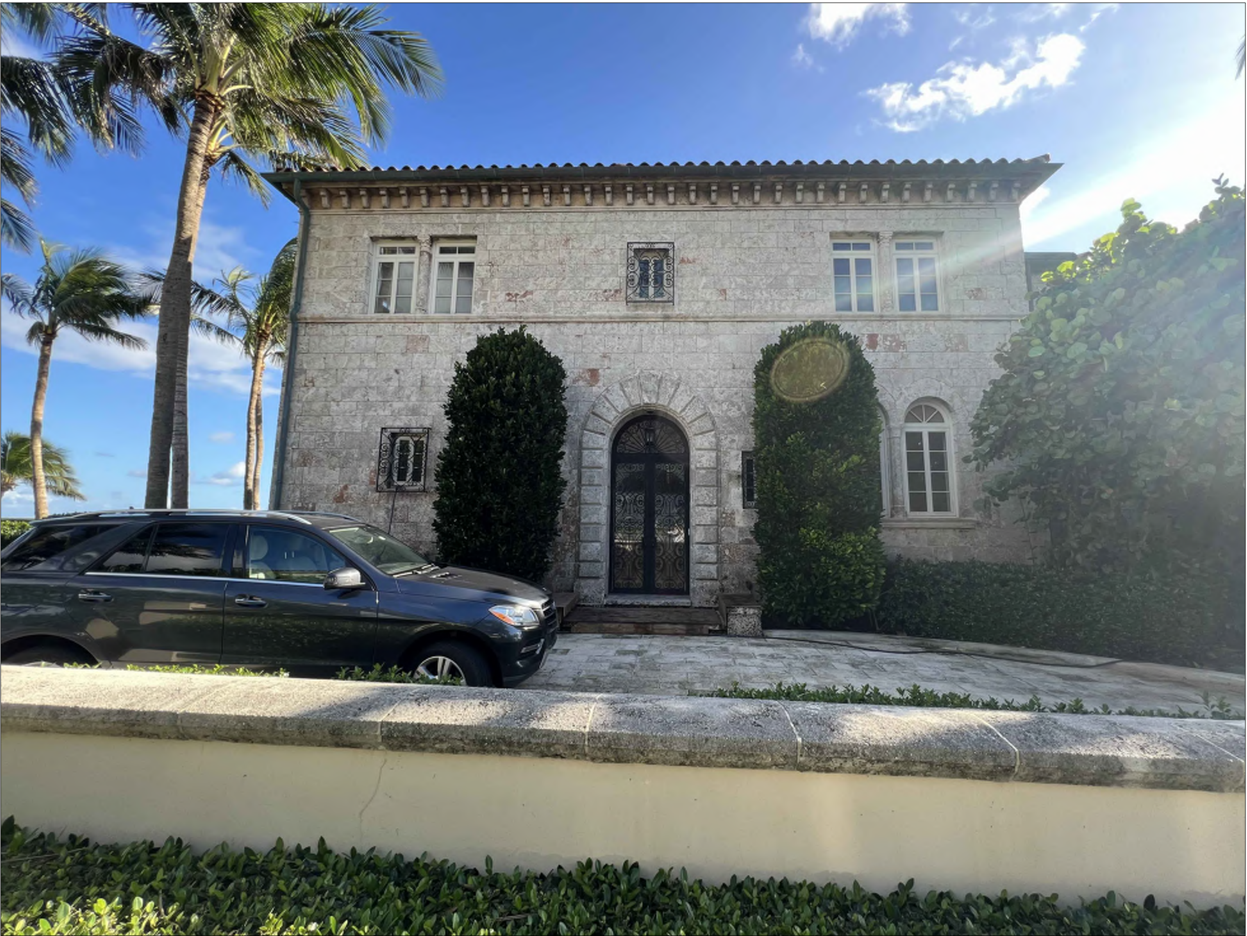
930 S Ocean Blvd -From Via Bellaria (Subject Property)
