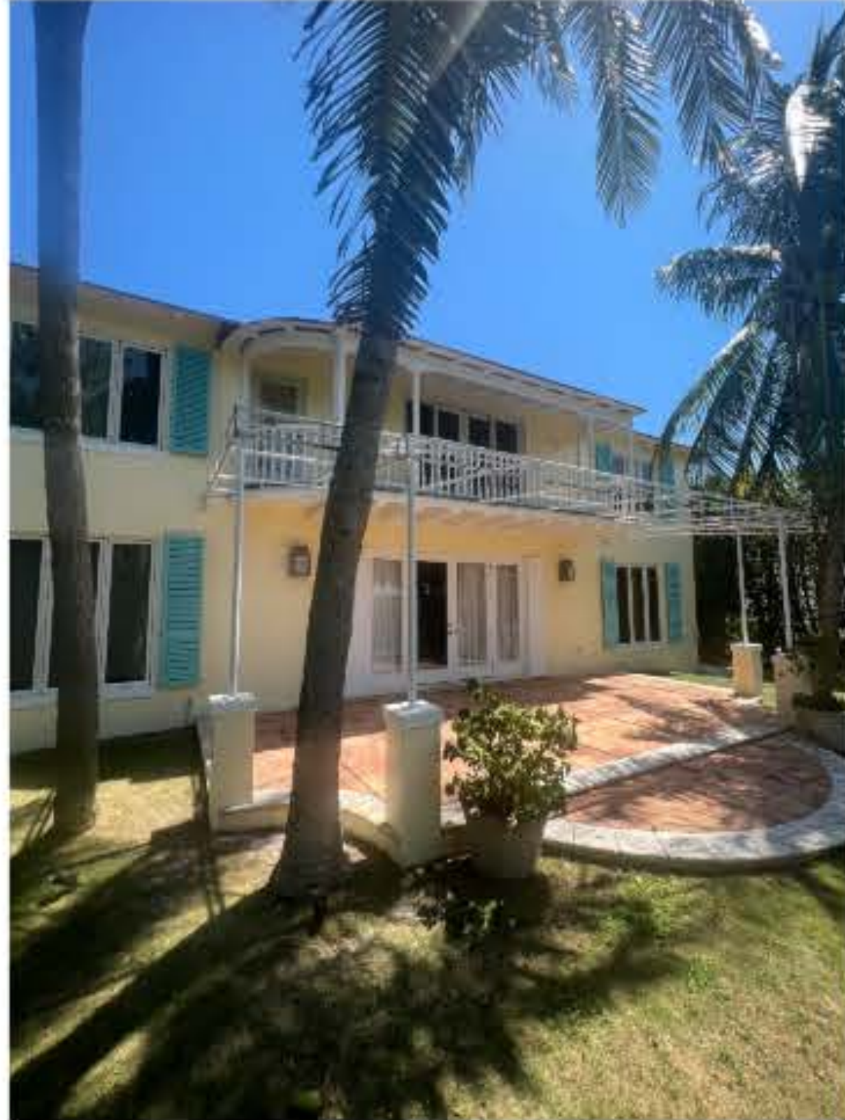
West Facade & Existing Terrace
