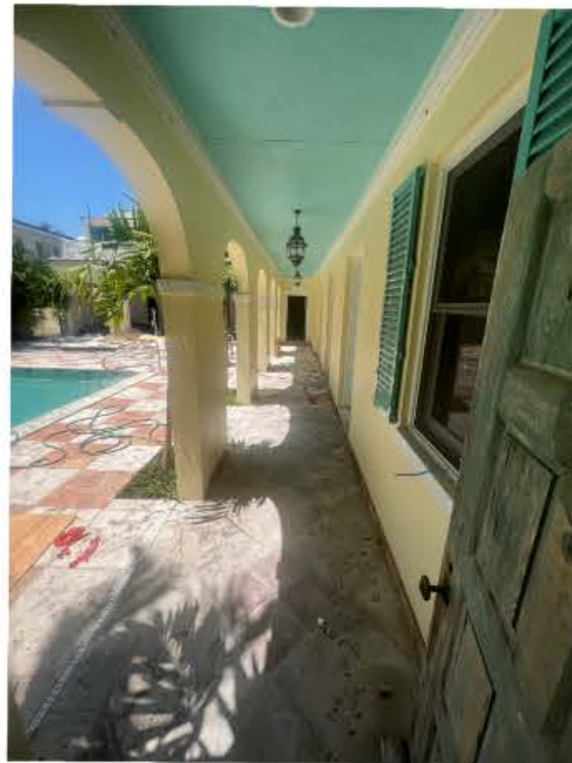
Covered loggia to front door
