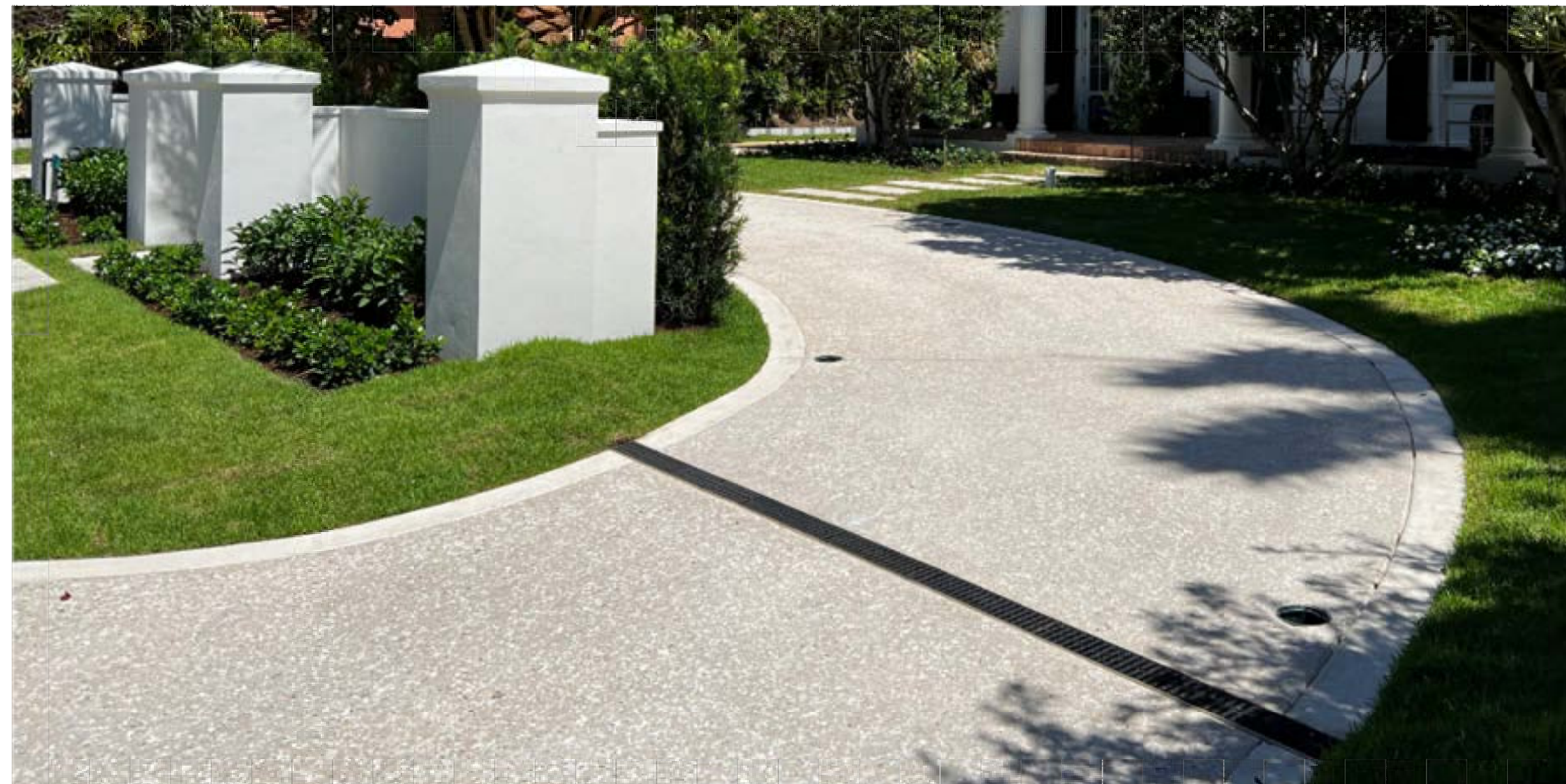
Tabby Motor Court: Textured center with smooth outer band. Concrete to match “shell” stone color
