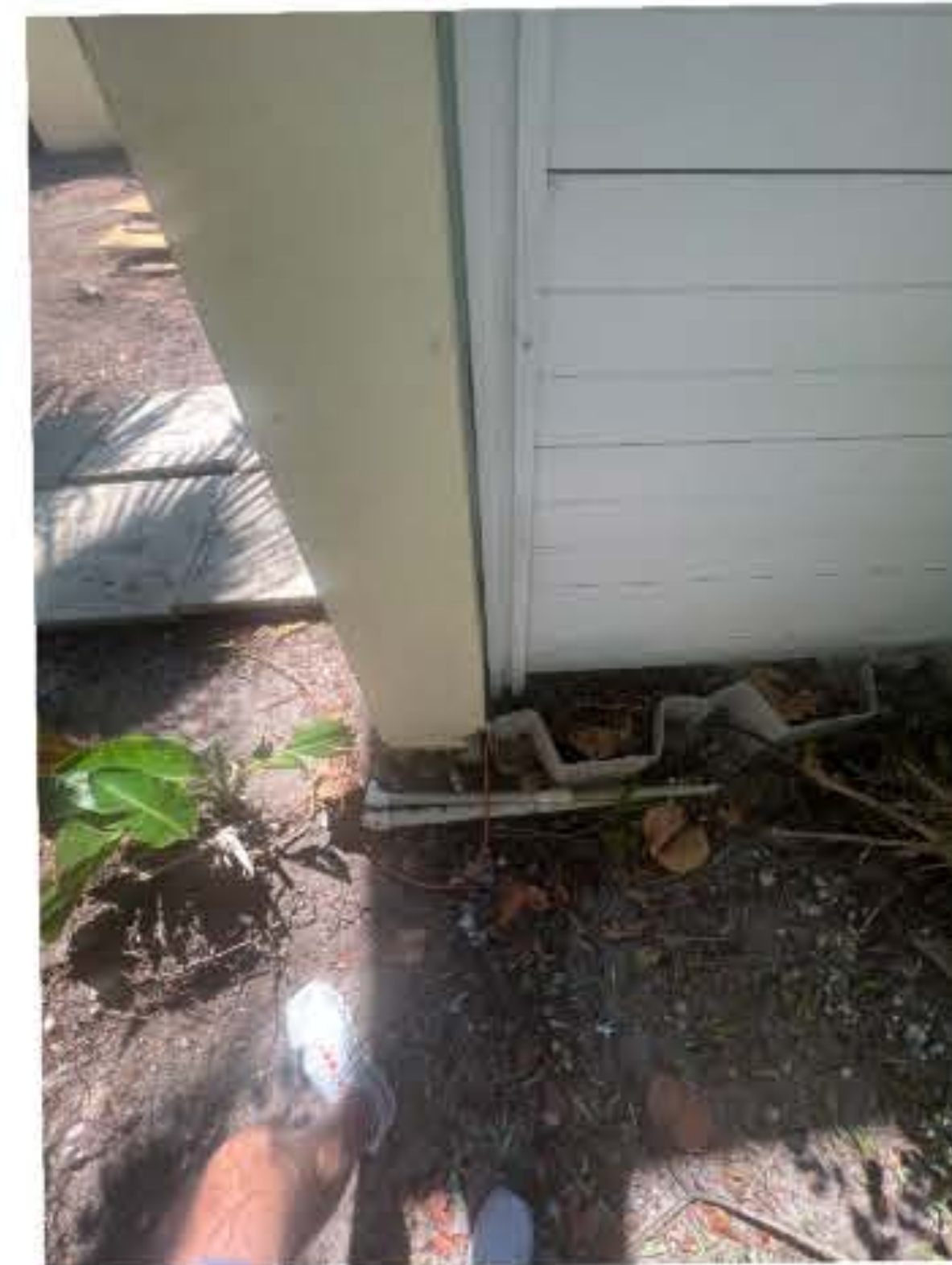
Exposed pipes, drainage walls and panels along Palmo
