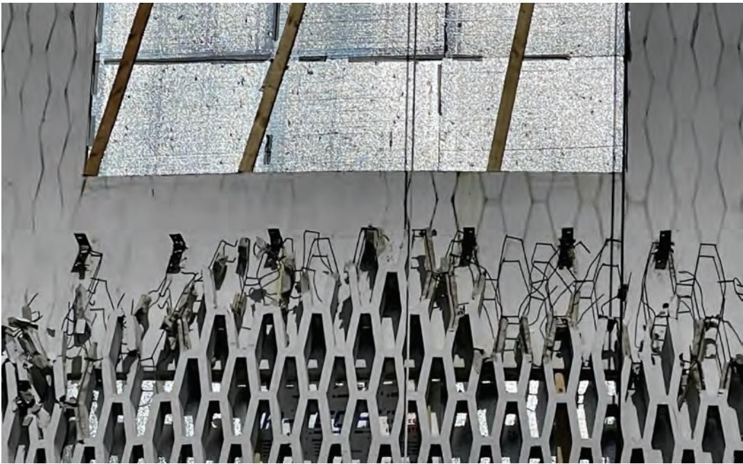
VIEWS OF CONCRETE SCREEN WALL REMOVAL
