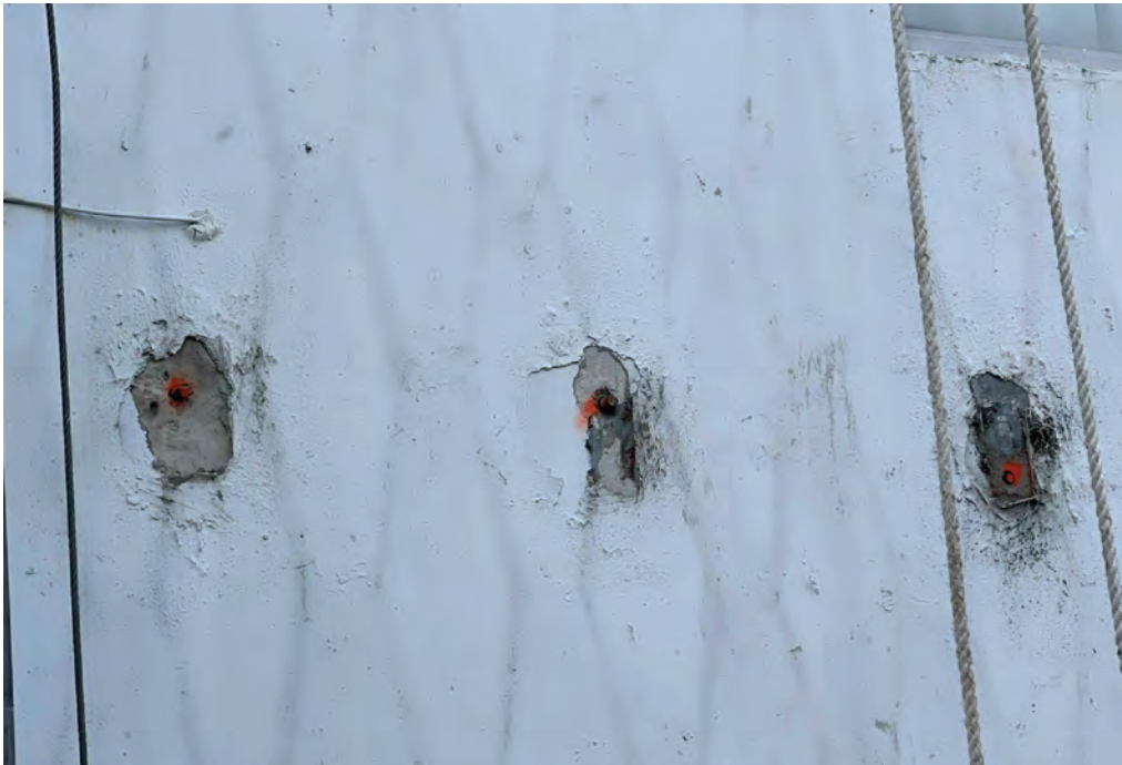
VIEWS OF CONCRETE SCREEN WALL SUPPORT POINTS
