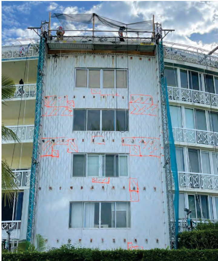
VIEWS OF CONCRETE SCREEN WALL REMOVAL
