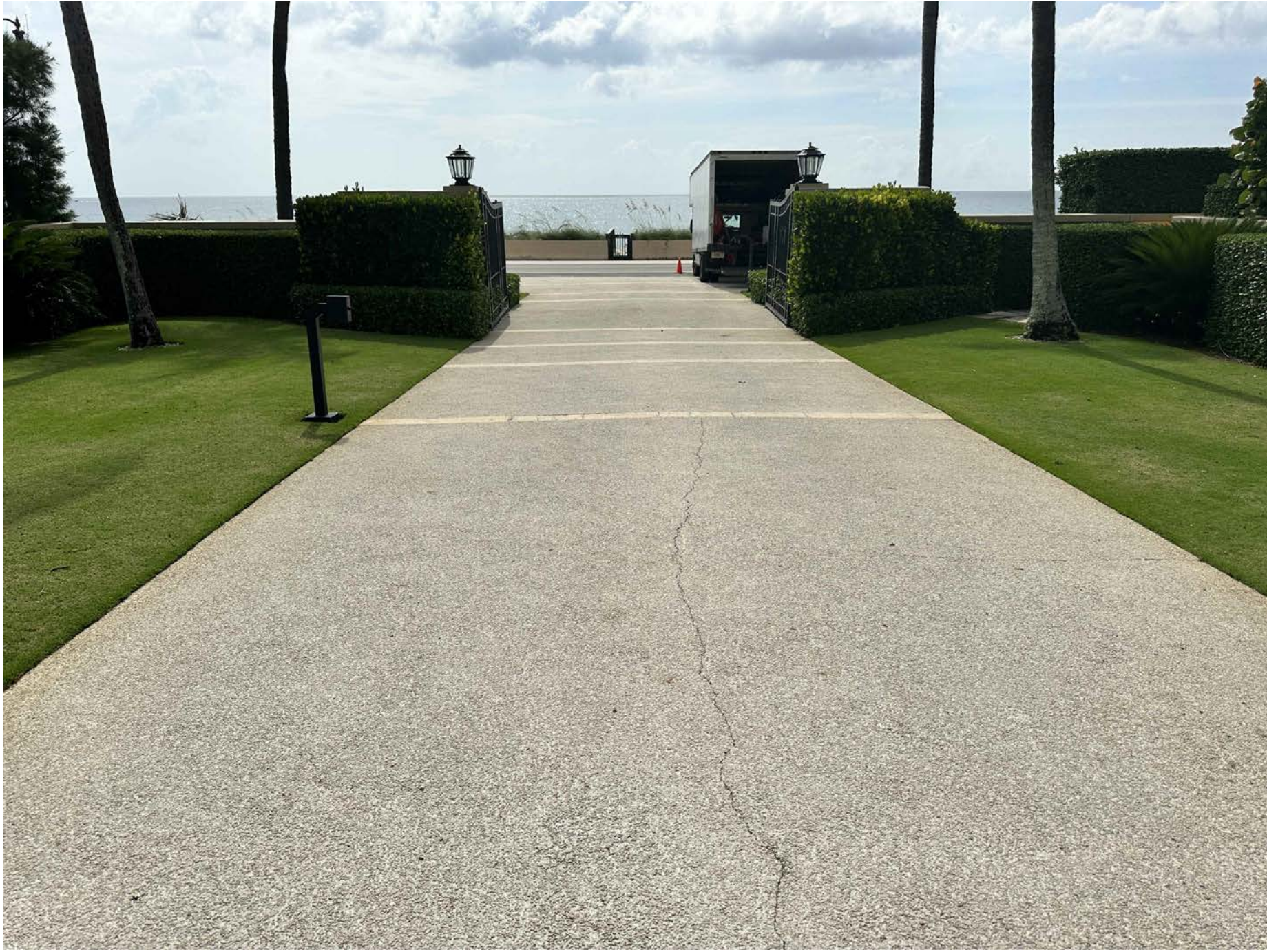
PHOTO 2: DRIVE WAY ENTRY AREA
