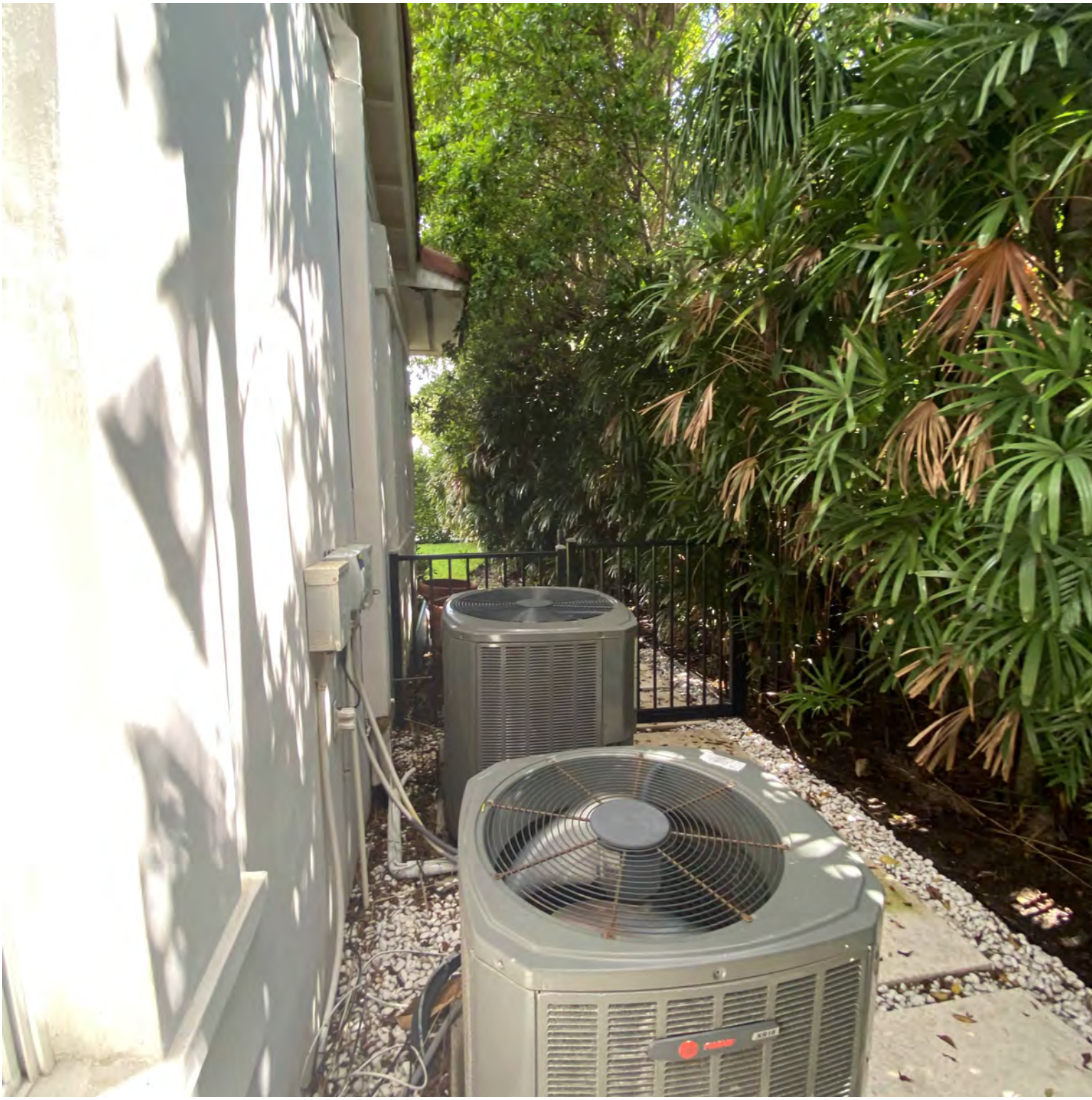
View to Existing East Yard
