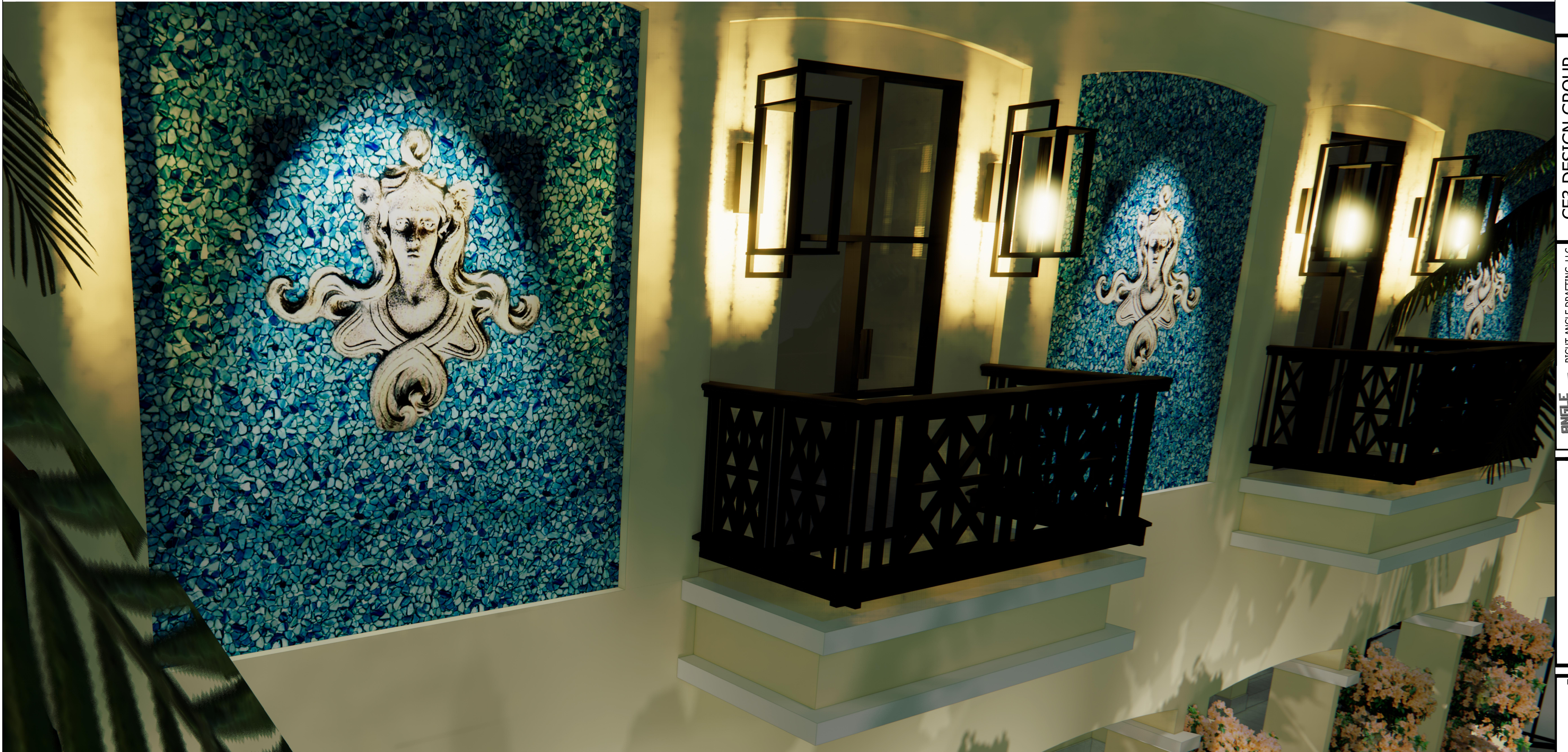
CLOSE-UP OF BALCONIES AT SOUTH SIDE OF BUILDING A
