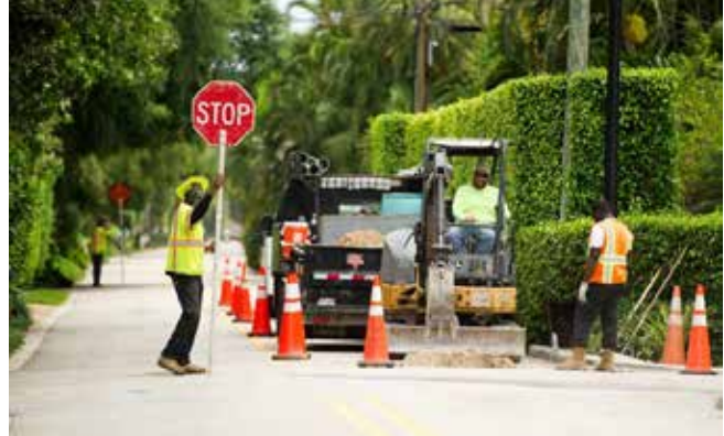
Workers Installing Underground Utilities
