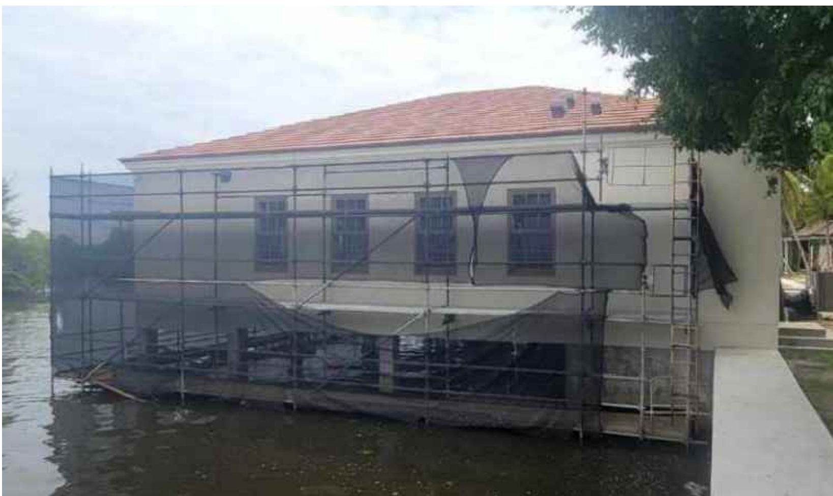
4. EXISTING BOAT HOUSE LOOKING NORTH
