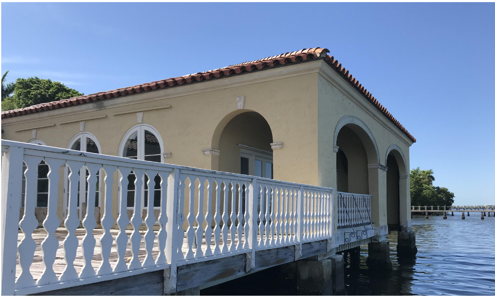
6. EXISTING BOAT HOUSE LOOKING SOUTHEAST
