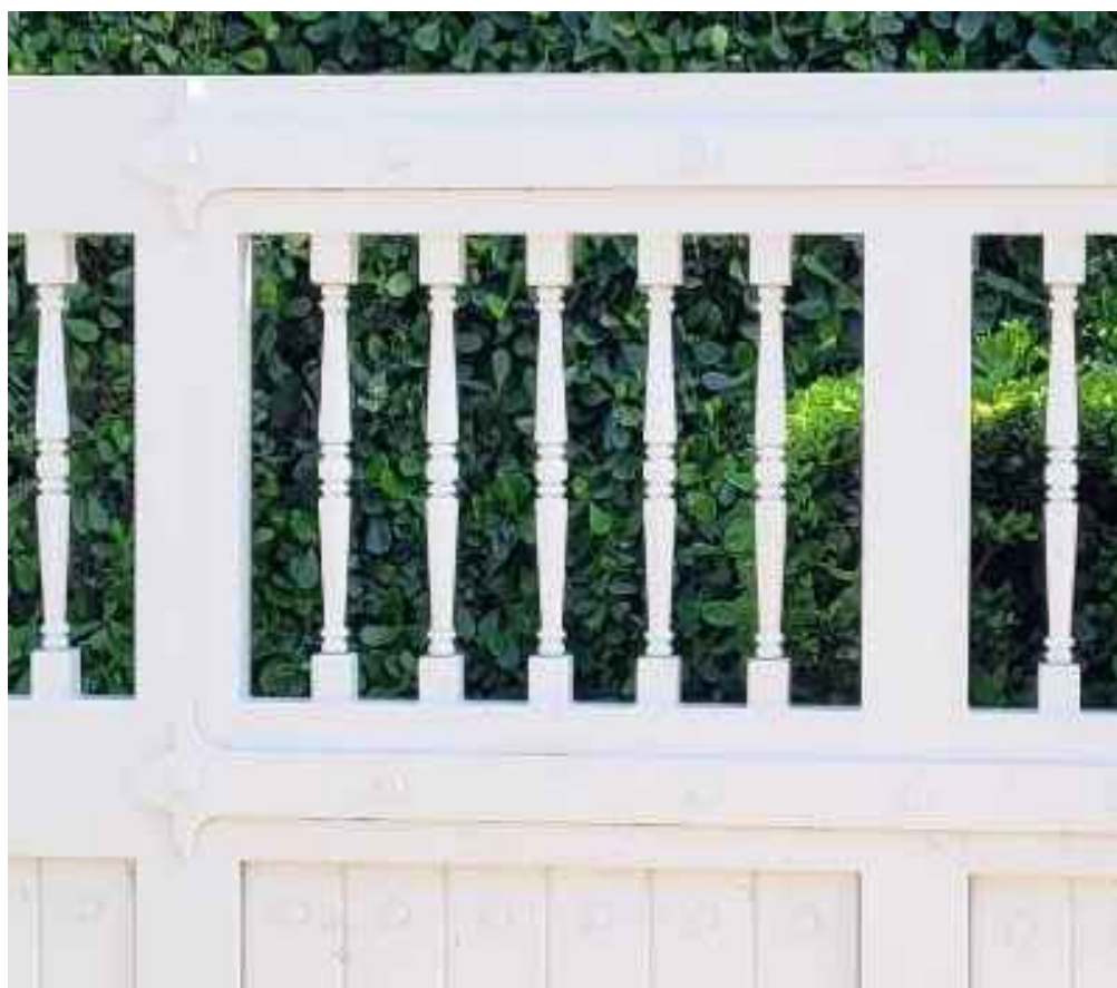
EXISTING GATE AT MAIN HOUSE
