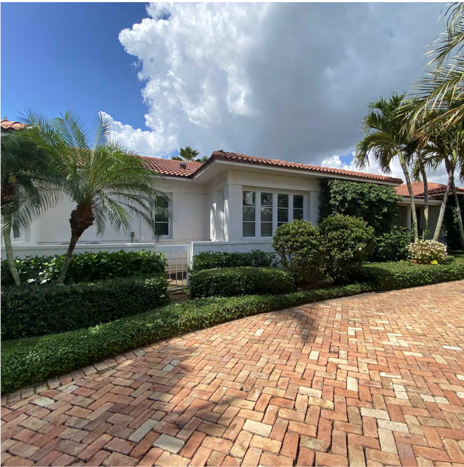
View to Existing Front Facade
