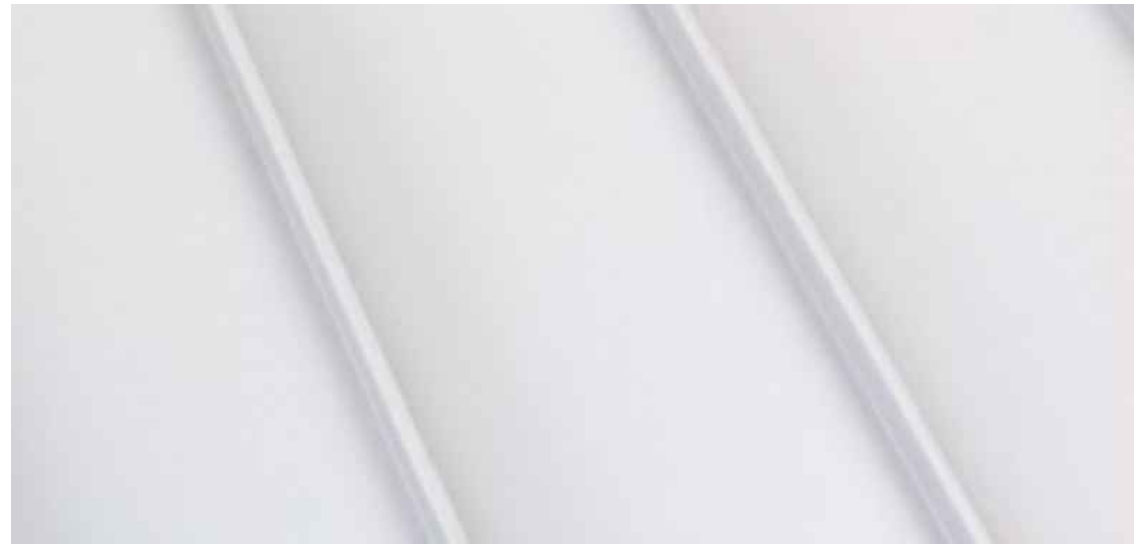
LOW SLOPE ROOF
