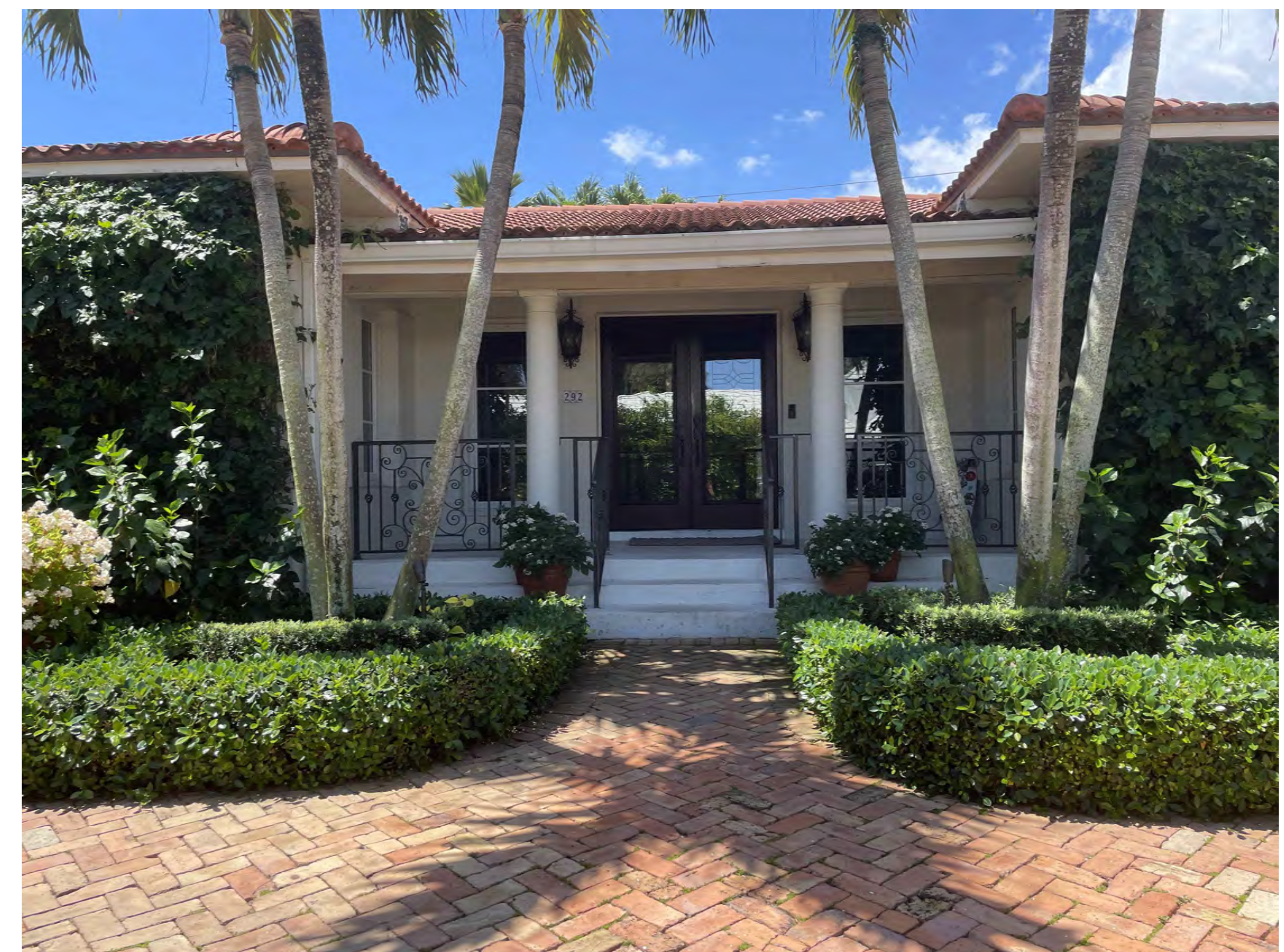
3- EXISTING COVERED ENTRY AT SOUTH ELEVATION
