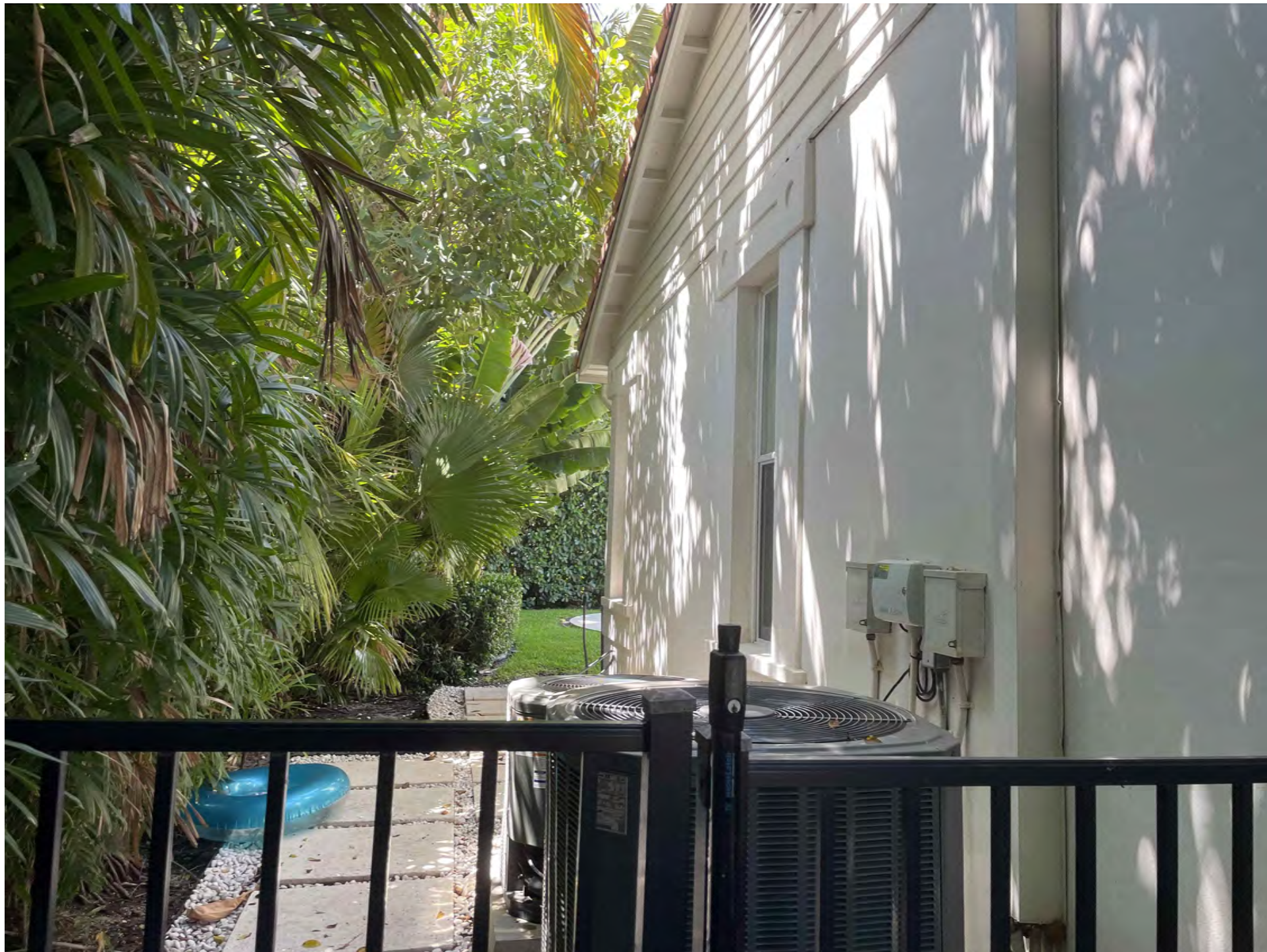
3- EXISTING EAST SIDE YARD
