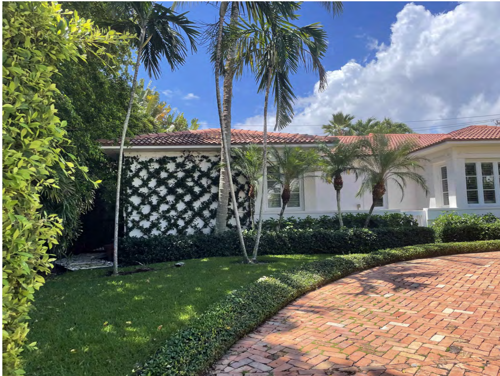
1- EXISTING SOUTH ELEVATION AT EAST SIDE YARD
