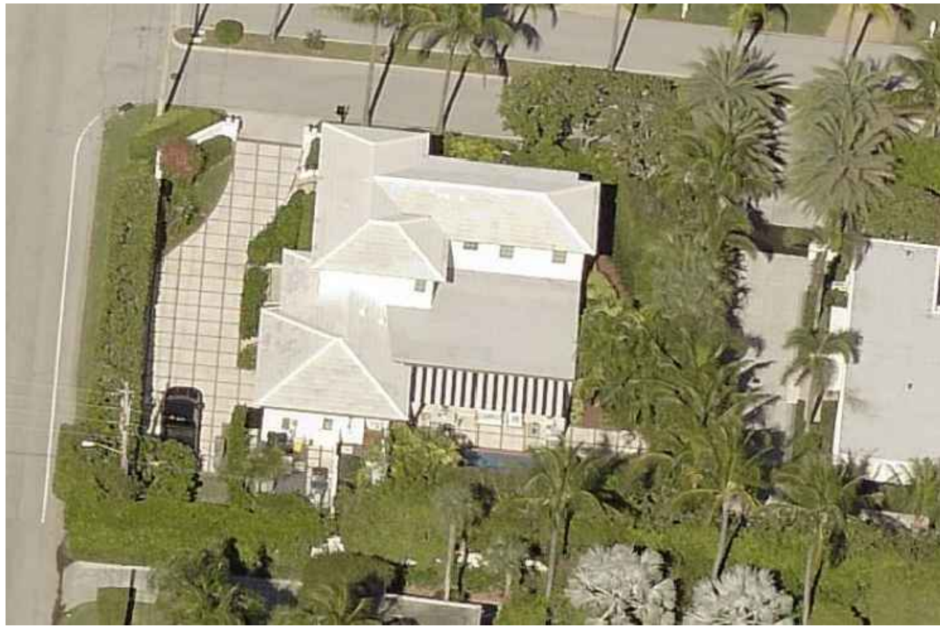
South West Aerial View
